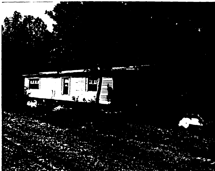
PHOTO 18: Typical Dwelling Downstream of Dam
