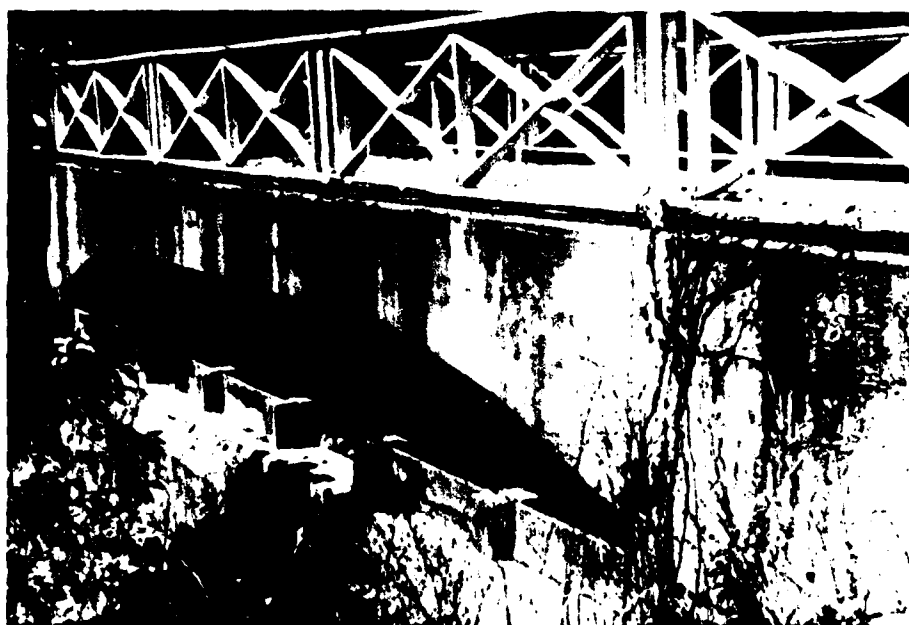
NO. 5: SPILLWAY WEIR AND BRIDGE
