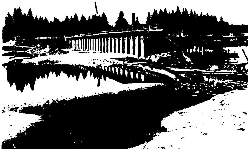
Figure 6. Failure of 14 piers and left abutment at Leech Lake Dam
