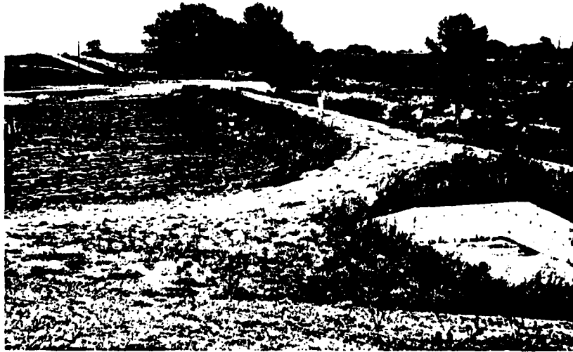
Photo 1 - View across spillway and along crest taken at right abutment.
