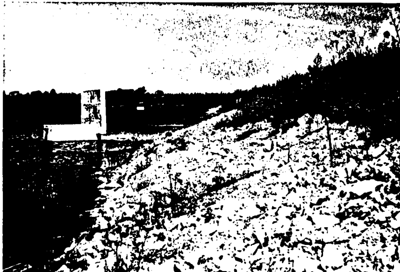
Photo 8 - Picture of drop inlet structure for service spillway.
