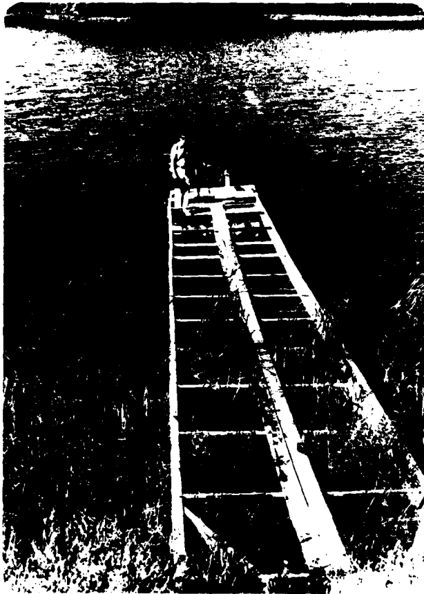
Photo 7 - Picture of intake structure and hoist for water supply piping.
