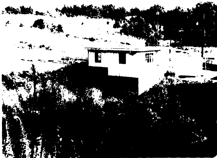
Photo 8 - Picture of water supply pump house.
