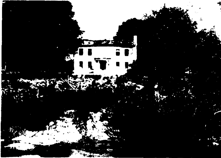
Photo 15 - View of a dwelling in the downstream hazard zone looking across Joachim Creek.
