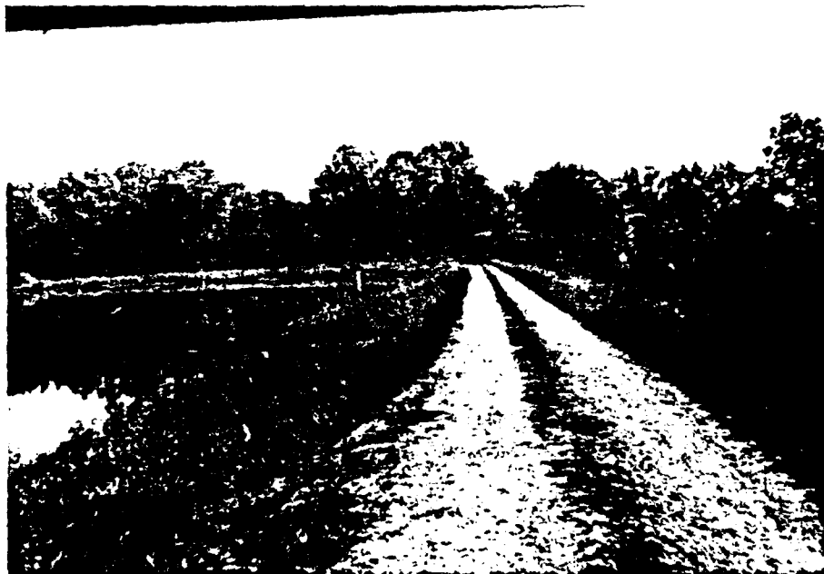
PHOTO 2 Crest of Dam
