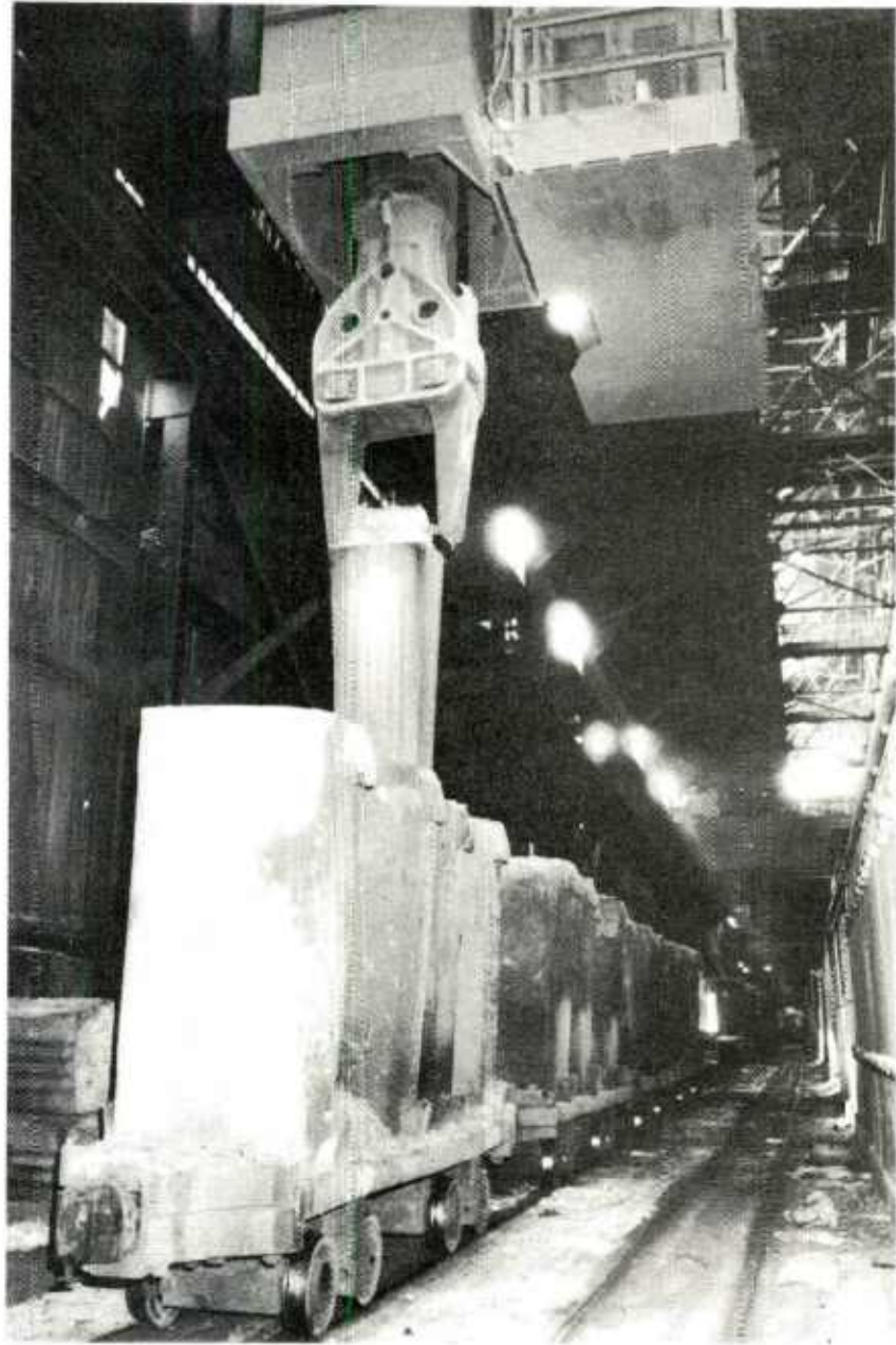
Figure B15. Preparing to charge ingots into soaking pits
