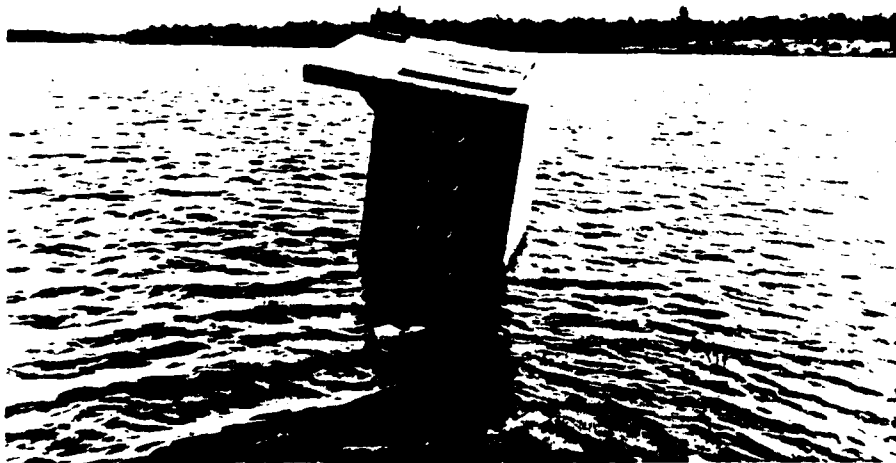
PHOTO NO. 13 OUTLET TOWER FROM SOUTH
