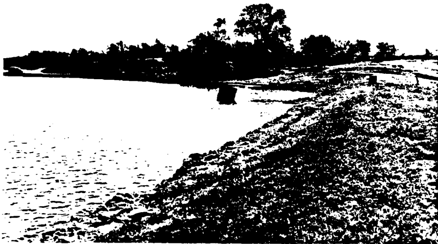
PHOTO NO. 12 UPSTREAM FACE AND OUTLET TOWER FROM WEST
