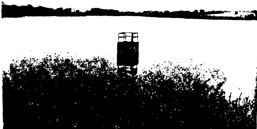
PHOTO NO. 5 GATE TOWER FROM CENTERLINE OF DAM LOOKING UPSTREAM.
