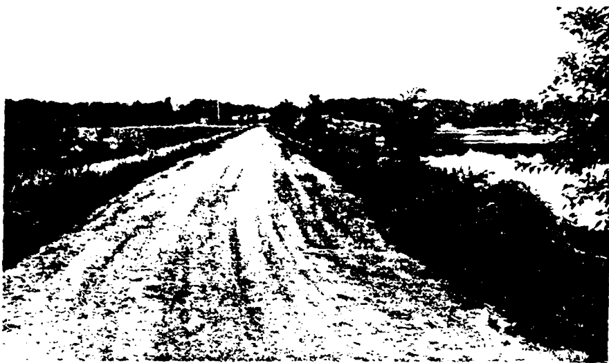
PHOTO NO. 2 TOP OF DAM. LOOKING WEST FROM EAST END.
