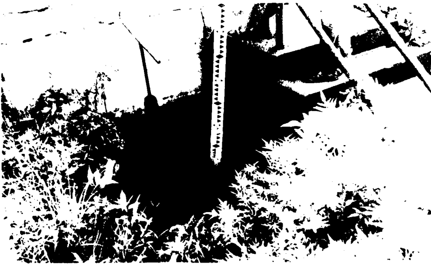
PHOTO. NO. 6 POND AND BOIL UNDER PUMPHOUSE STEP. DOWNSTREAM FROM C STA. 4+20±.
