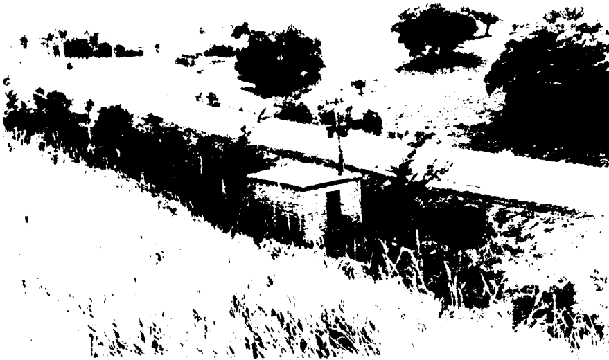
PHOTO. NO. 11 PUMPHOUSE FROM CENTERLINE STA. 4+20.
