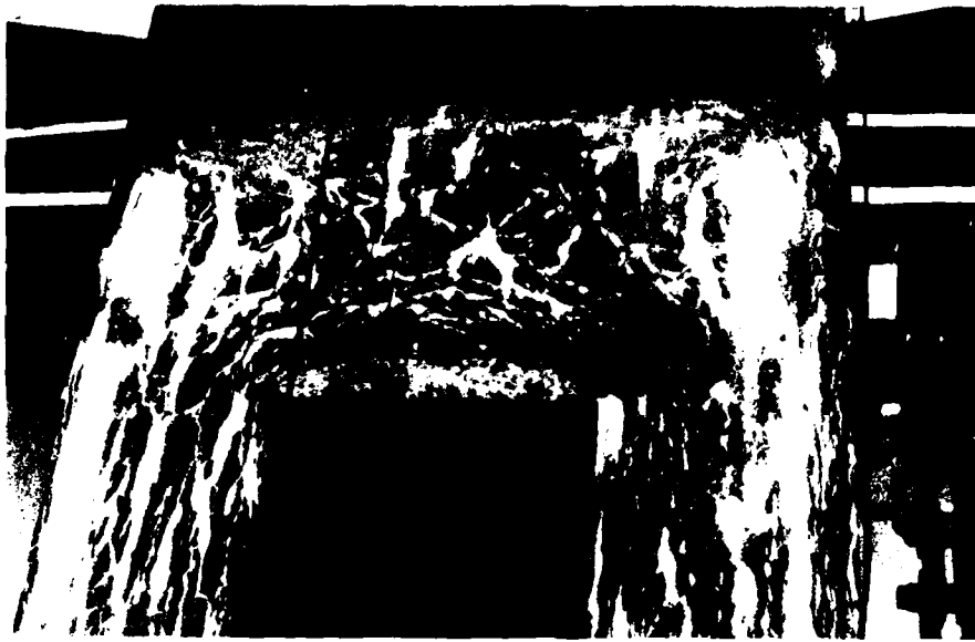
Photo 3. Looking at downstream faces of service bridge support columns, pier No. 9. Typical crack pattern and exudation of severe deterioration
