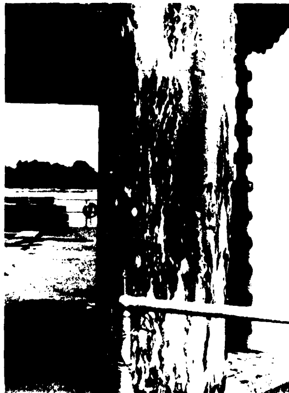
Photo 3. Looking at downstream faces of service bridge support columns, pier No. 9. Typical crack pattern and exudation of severe deterioration
