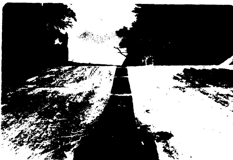
DRAINAGE CHANNEL FROM UPPER PLUNGE POOL TO EXIT CHANNEL
