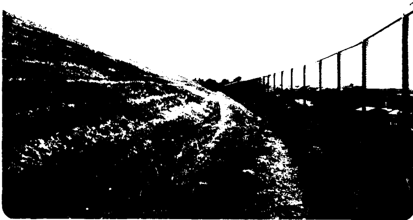
4. Easterly slope of embankment.
