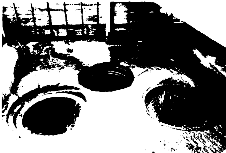
Three Wells within Drop Inlet Structure Leading to Spillway Outlet Pipes; Note Cracked Concrete
