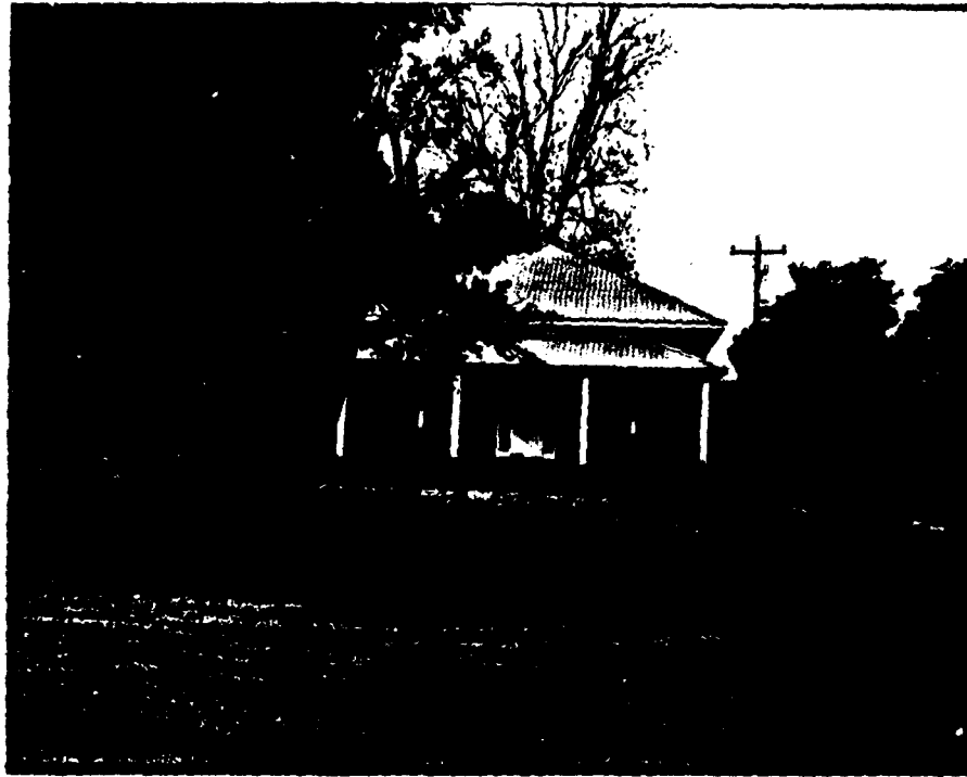
PHOTO 15: Uninhabited Dwelling Downstream of Dam .
