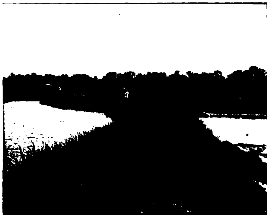
PHOTO 10: Guide Levee between Farm Pond and Lagoon
