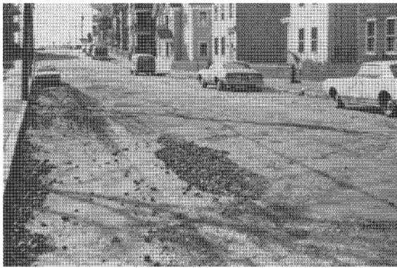
Macadam pavement unravels dramatically when water enters
