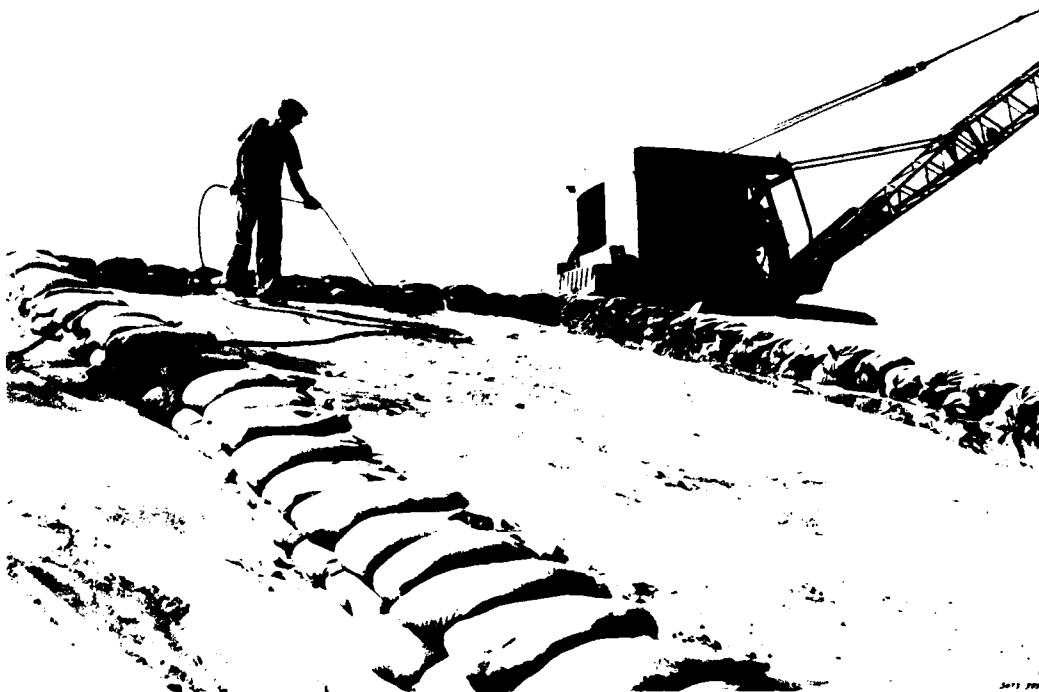
Photo 52. Form constructed of bagged concrete mix on MESL Item 6; bags being sprayed with water to cure mix in bags
