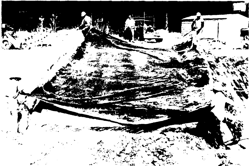
Photo 20. "Blanket" of material being placed over the soil
