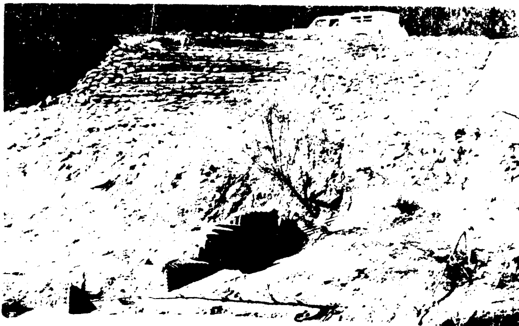
Photo 57. Items 7 and 8 - Riprap on Bidim C-38 filter fabric and T15 membrane stepped section
