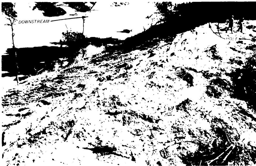
Photo 40. View of bank area with vegetation removed (note hole in bank). This area of bank selected for stepped MESL item (Item 8)
