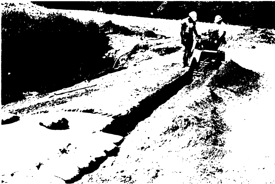
Photo 14. Construction of anchor ditch
