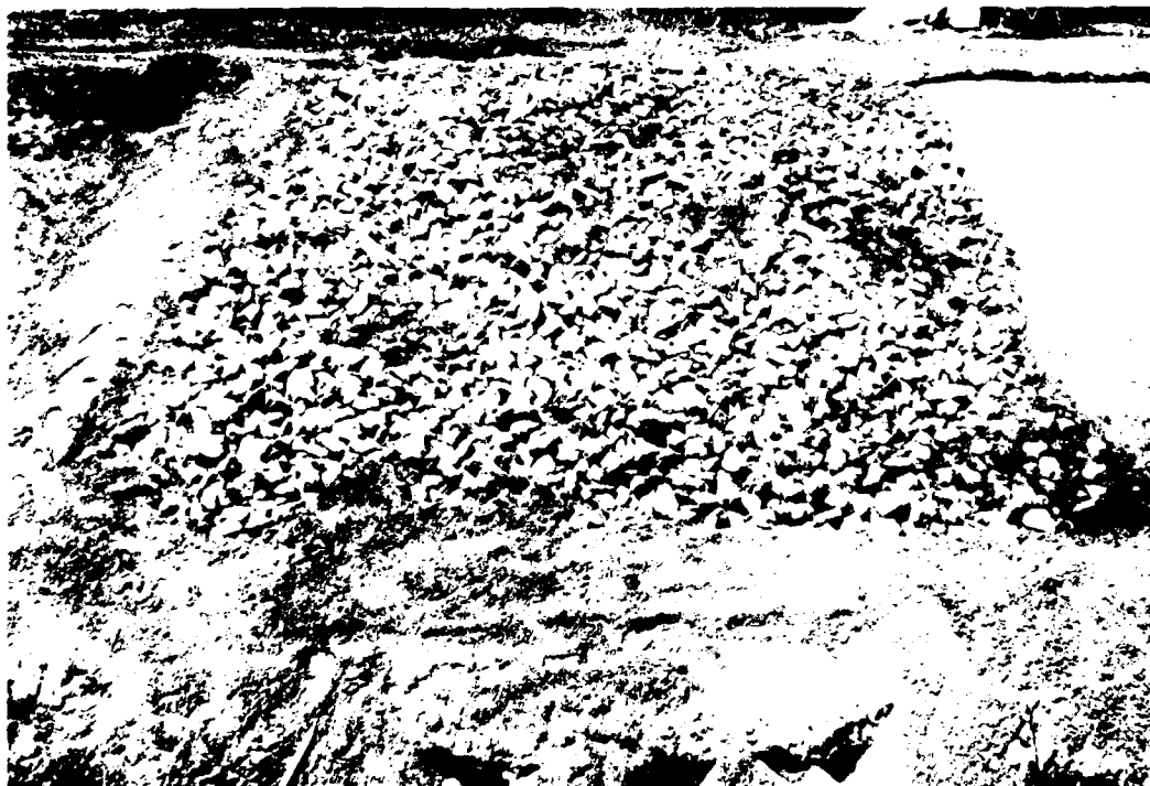
Photo 32. Item 7 - Bidim C-34 fabric covered with riprap
