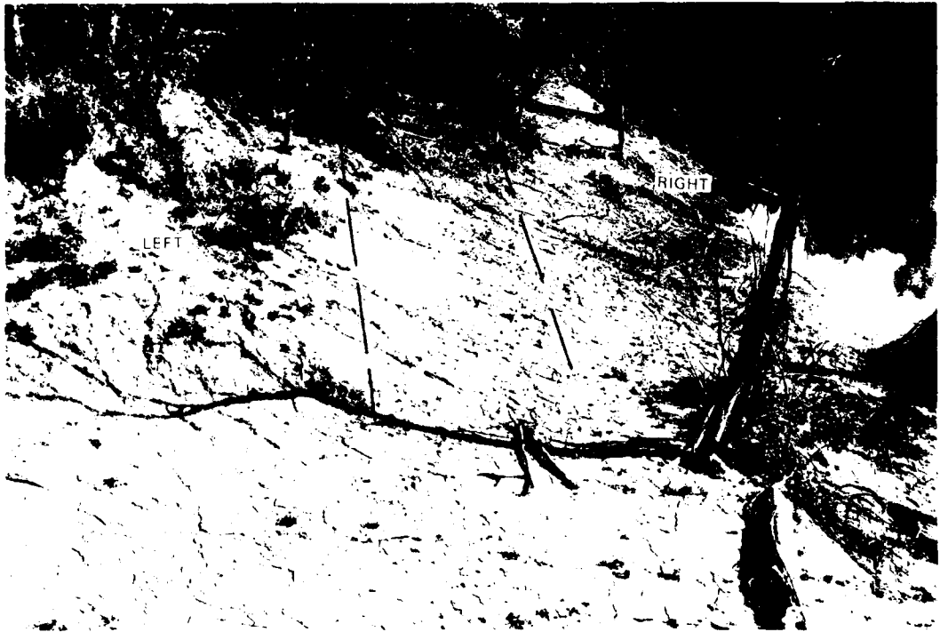
Photo 84. View of riverbank downstream of test area where sliding and slumping occurred as a result of the sudden drops in the water level of the river
