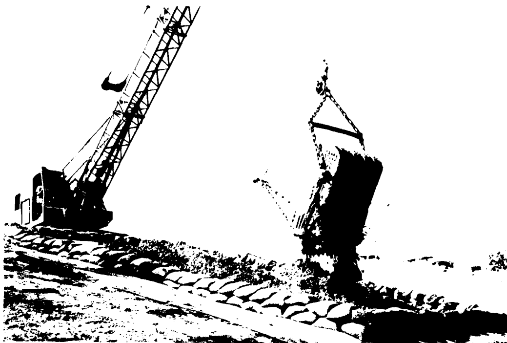
Photo 53. Backfill material being placed in form of MESL Item 6
