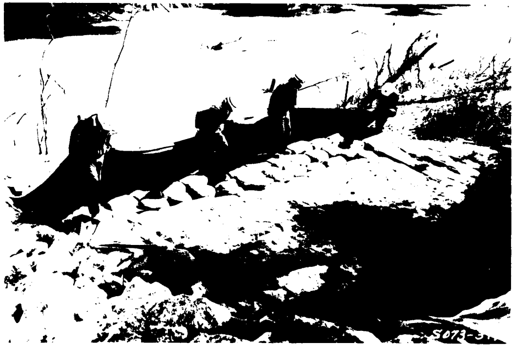
Photo 56. Placement of top sheet of membrane on the first step of Item 8
