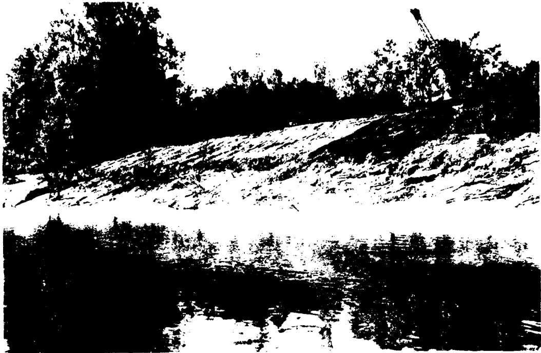
Photo 41. Shaped test site and excavation of bank for Item 1
