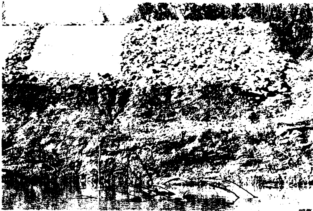
Photo 49. Items 1 and 2 - riprap on Bidim C-38 filter fabric and Hypalon 5x5 membrane
