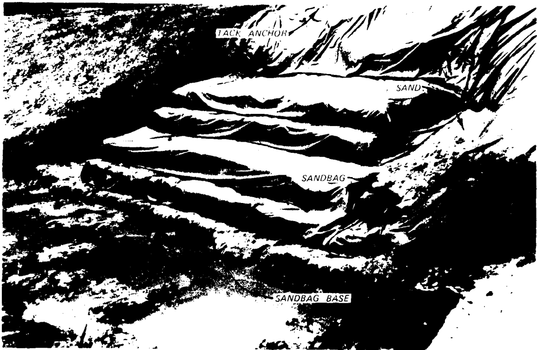
Photo 17. Completed steps of stepped MESL item
