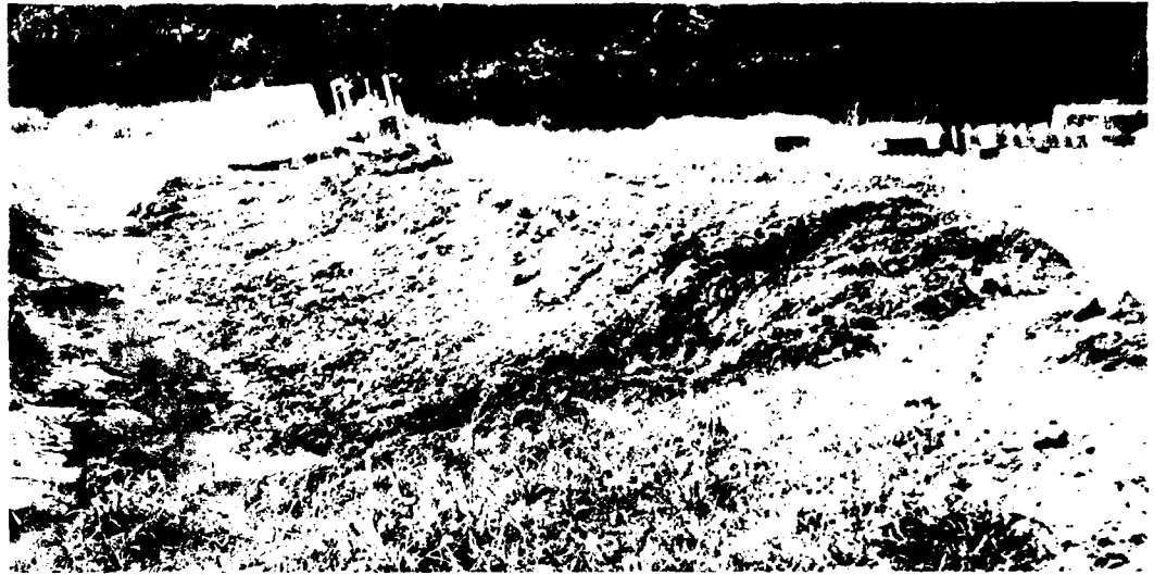
Photo 11. View (looking downstream) of D-4 dozer used to shape the bank of the test area
