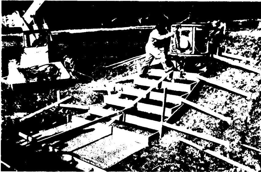
a. Placement of concrete
