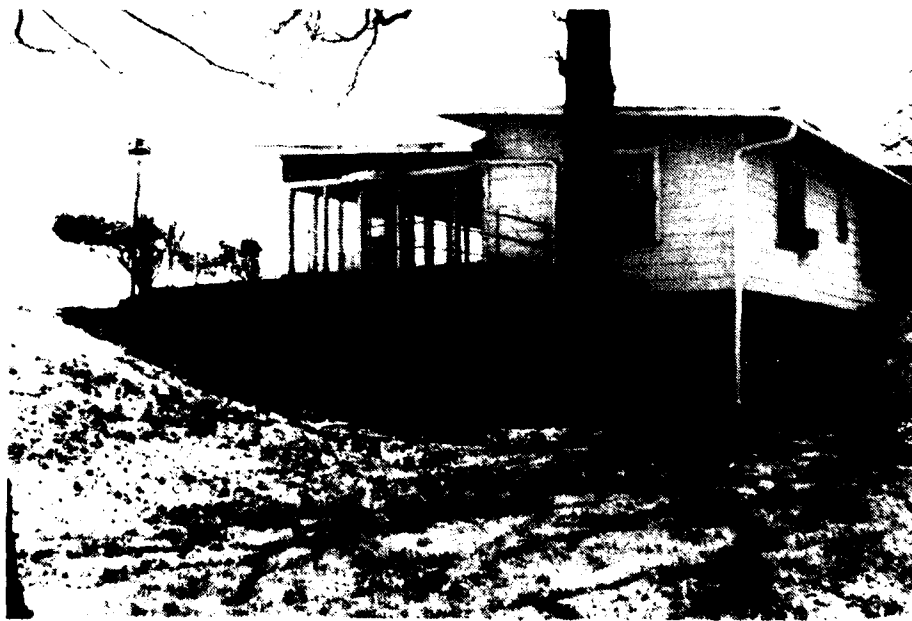
4. House with foundation and lower floor built into downstream slope of Nolan Dam.
