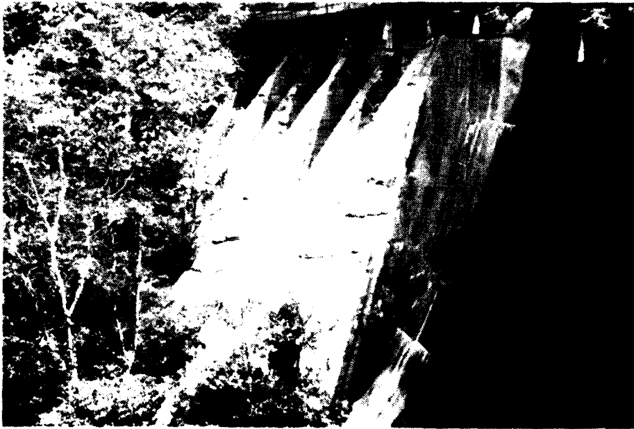
2. Downstream face of Cumberland Springs Dam. Note erosion of buttresses.
