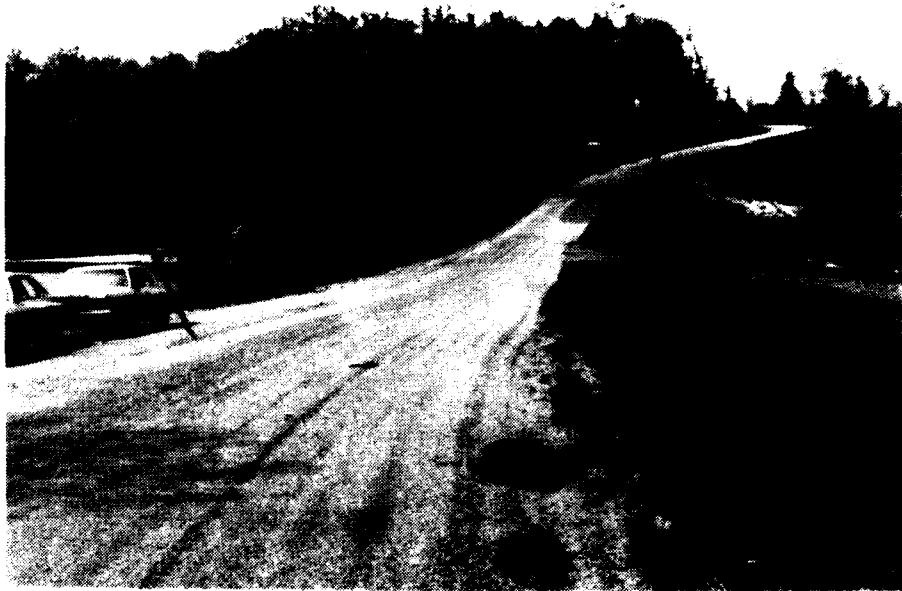
9. Low area at top of dam near left abutment used as emergency spillway.
