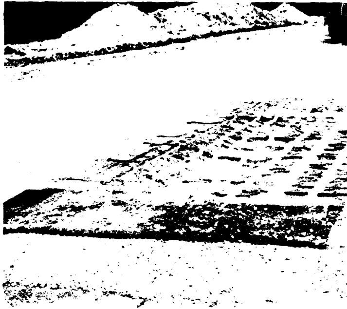
Photo 83. End of fabric rolled back to show condition of bottom surface after loss of bond
