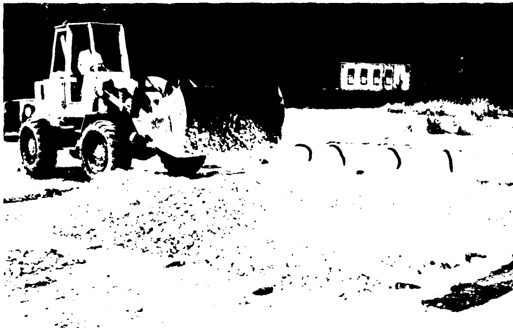
Photo 35. Front-end loader placing initial limestone over slotted plastic pipes in crater 2
