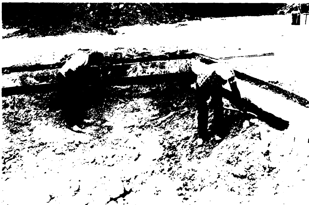
Photo 48. Undercut being excavated in north half of crater 4, prior to placement of reinforcement steel
