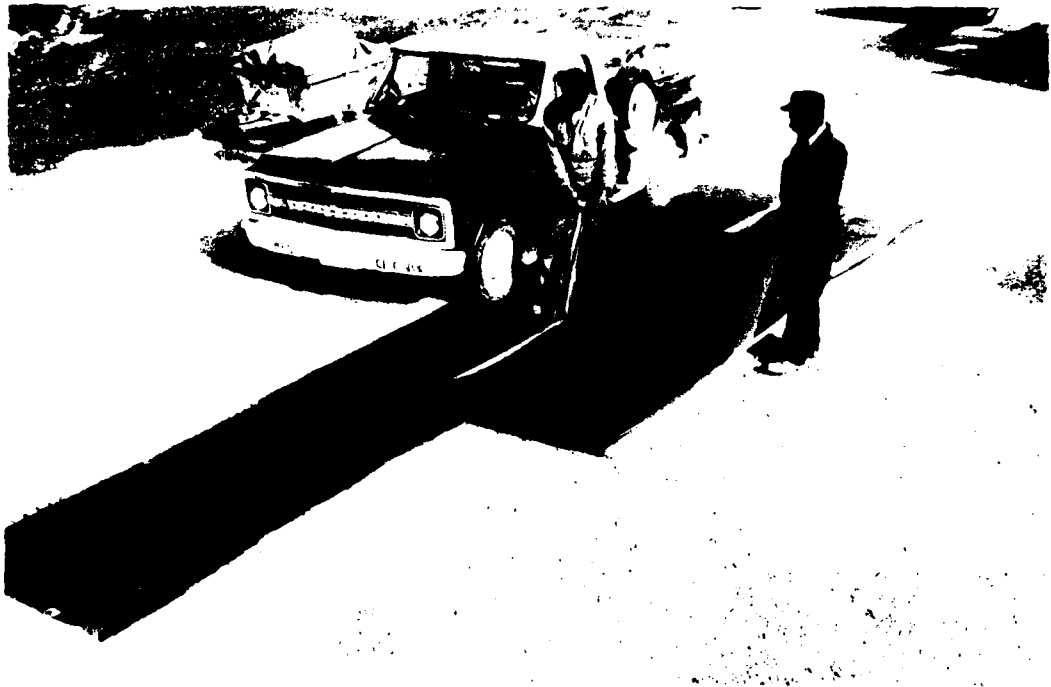
Photo 79. Asphaltic film being placed by hand over surface of limestone to keep individual limestone aggregates intact
