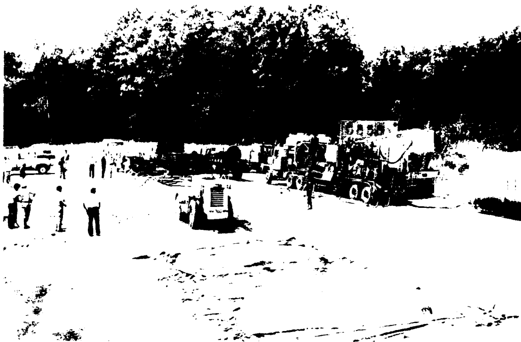
Photo 47. Vibratory steel-wheel roller compacting limestone in crater 3, while crater 2 (in background) is being filled with grout
