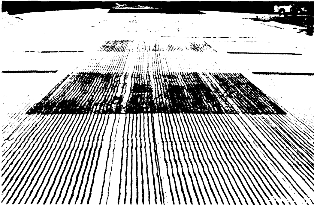
Photo 17. Asphalt emulsion sprayed on portland cement concrete as a tack coat prior to overlaying with asphaltic concrete
