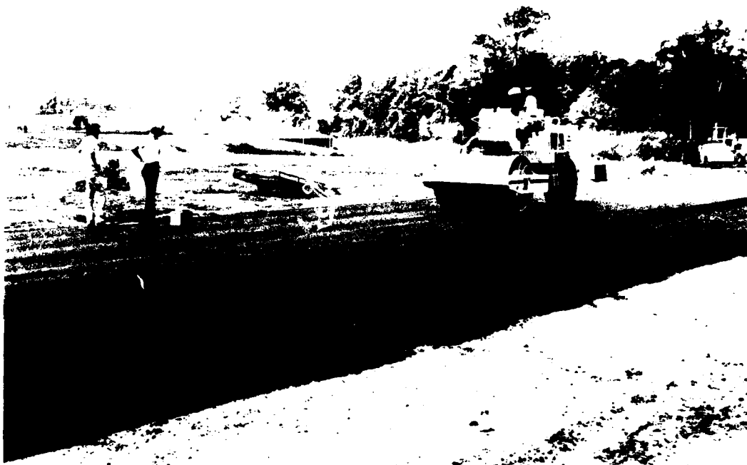
Photo 19. Vibratory steel-wheel roller compacting asphaltic concrete
