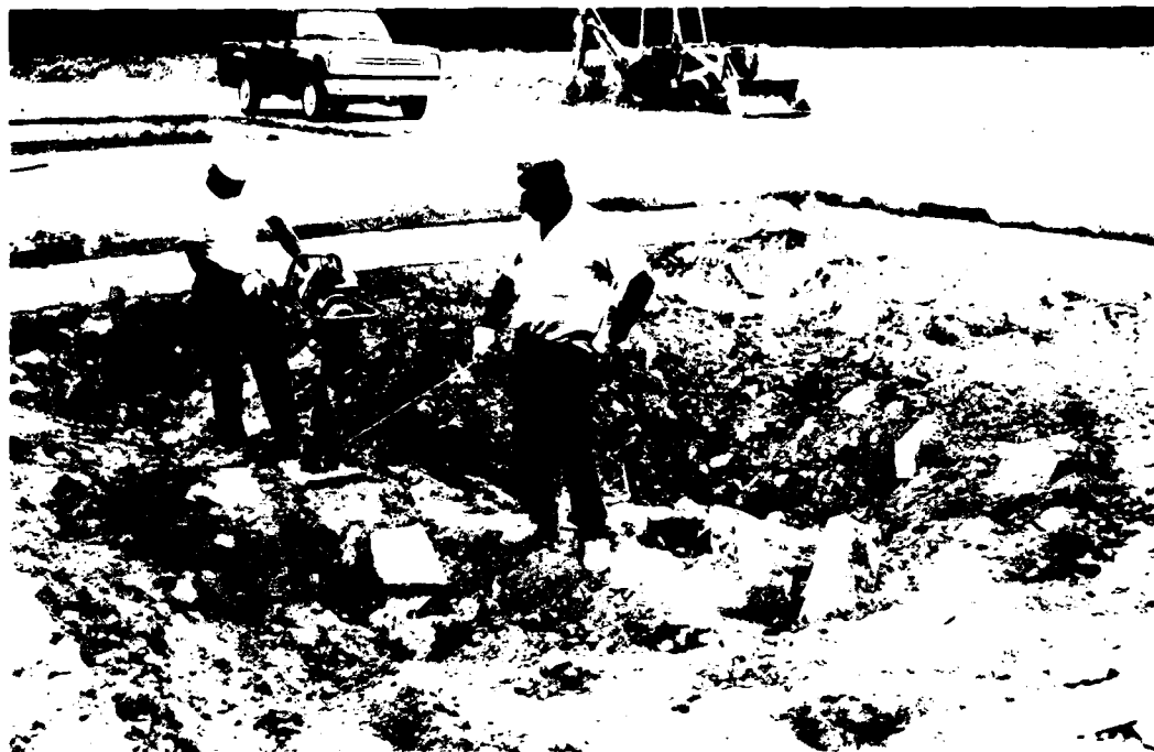
Photo 27. Rubble being compacted in crater 5
