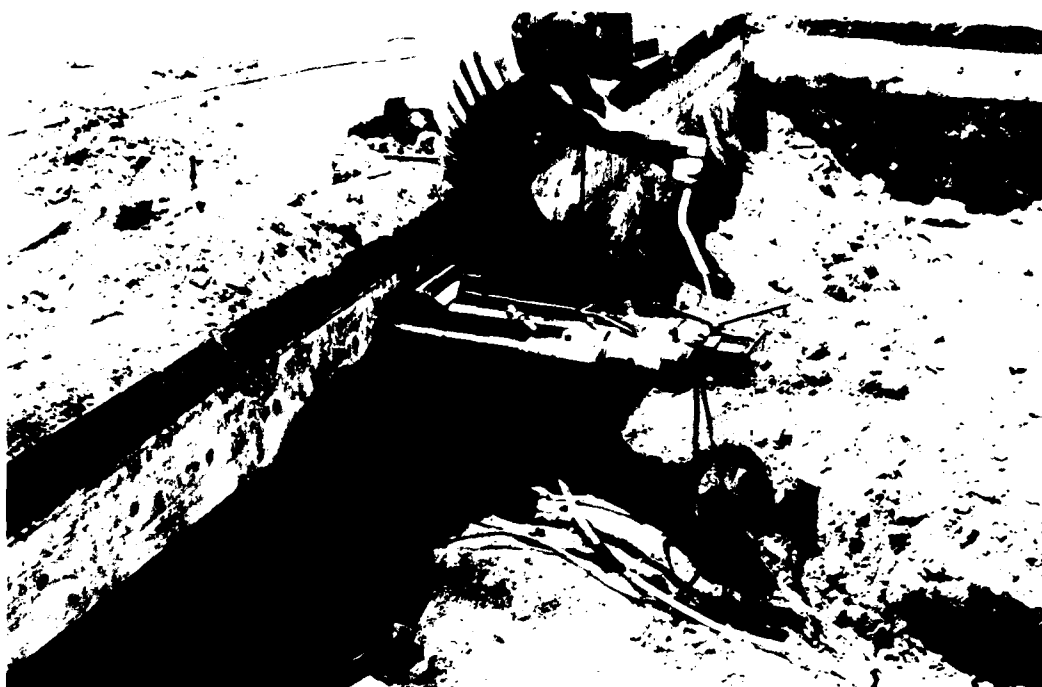
Photo 49. Drilling of 1-1/4-in. holes in existing vertical face of concrete slab for placement of steel dowels in south half of crater 4
