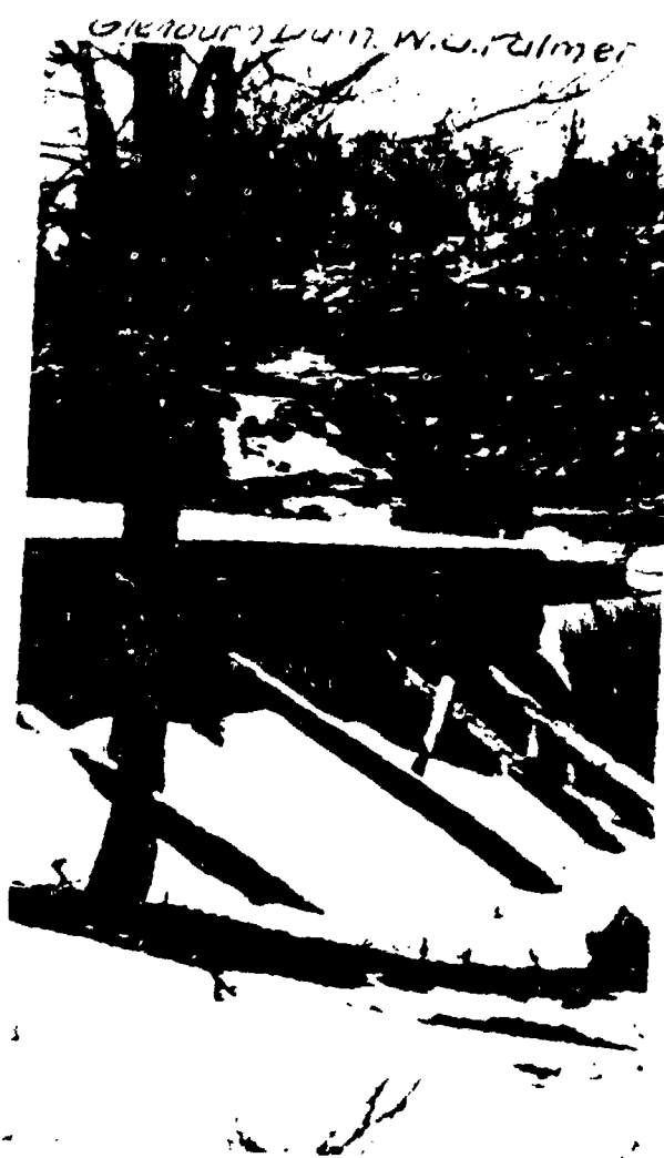
2. (1914 PHOTO) VIEW OF TEMPORARY SUPPORT OF RIGHT DRY STONE WALL
