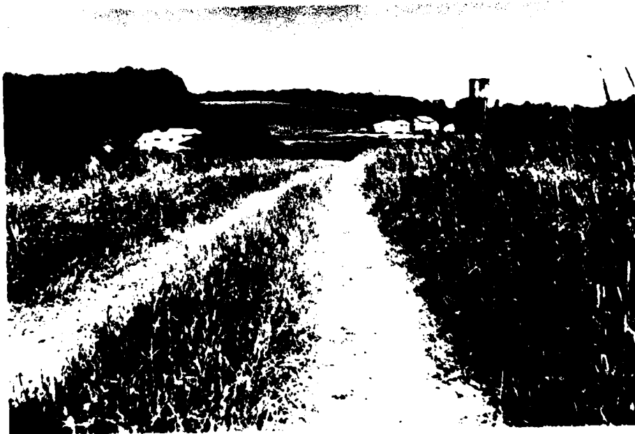
TOP OF DAM AND TIRE TRACKS
