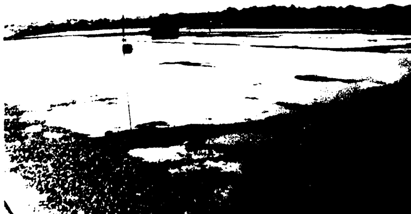
Figure 1. Ponds on the flat roof of the Reserve Center garage, June 1979.
