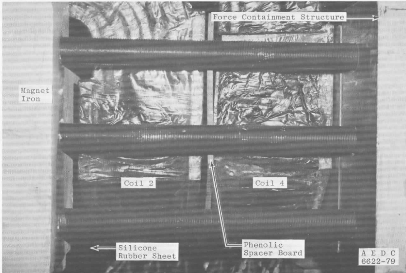
Figure 35. Nonuniform spacing between coils no. 2 and no. 4.
