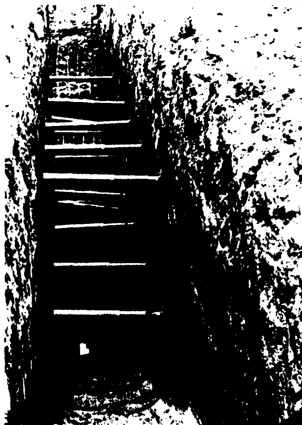
View of trench LD-T-9 with hydraulic shoring in place (Looking North).
