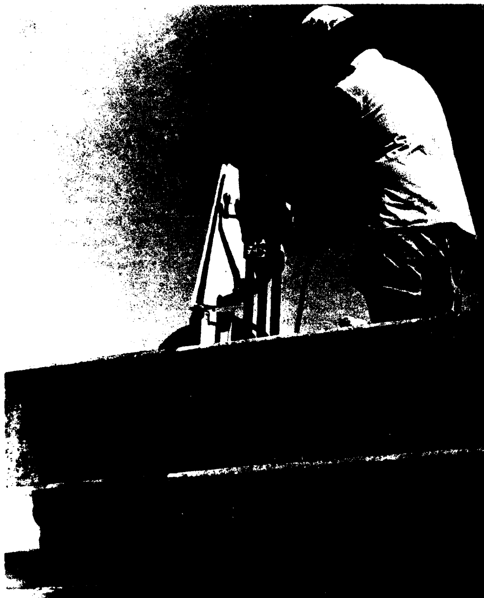
Figure 5. Bridge deck being cut with a rotary-action diamond saw (courtesy of Concrete Coring Company, Hawthorne, Calif.)
