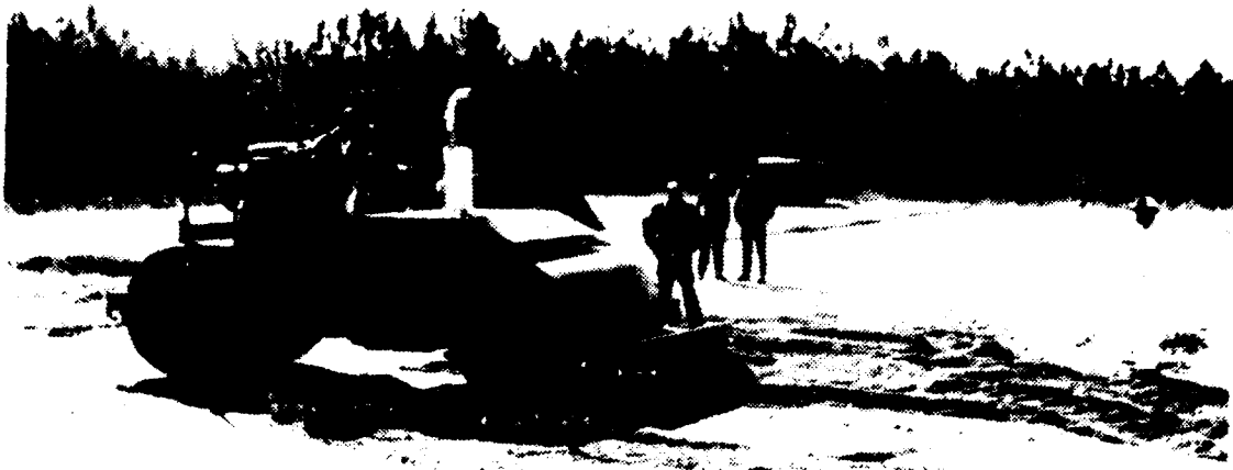
Figure 13. Pettibone C-44 Grading and Compacting
