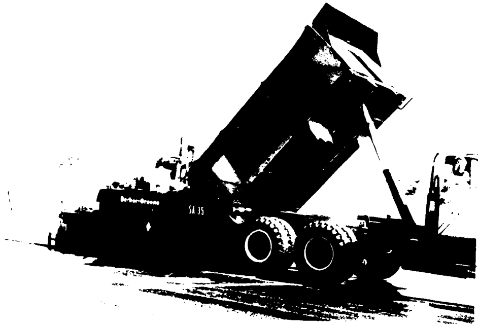
Figure 9. Finishing machine, Bituminous material.
