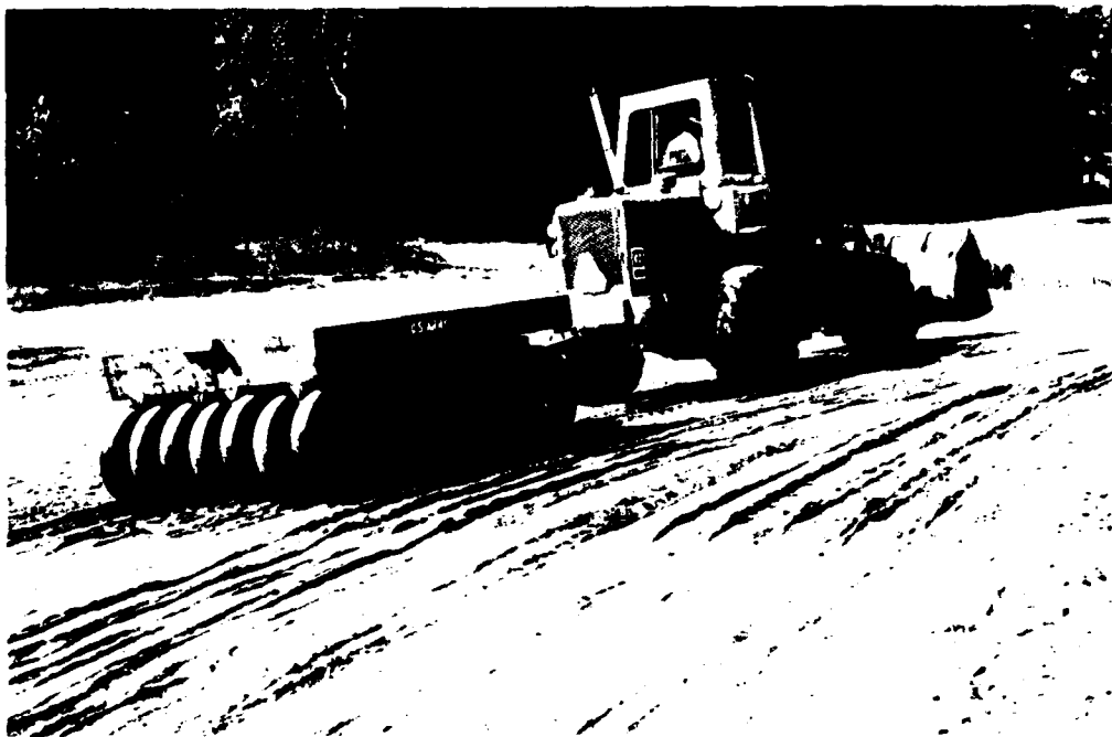
Photo 7. Rubber wheel roller used for compaction purposes
