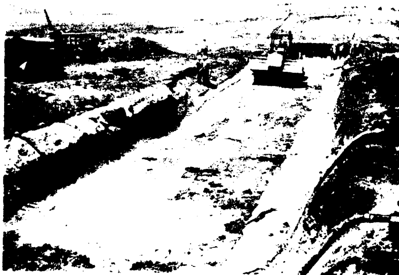
2. Melvern Lake, Construction Photo, Neg. No. 86612-6 (Placing impervious backfill in cutoff trench)
