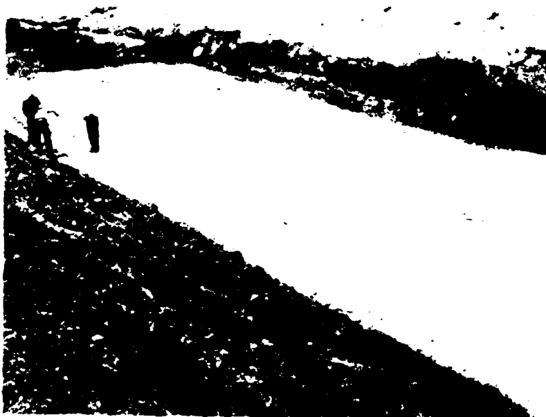
4. Melvern Lake, Construction Photo, Neg. No. 694-R1-23 (Impervious backfill in cutoff trench)
