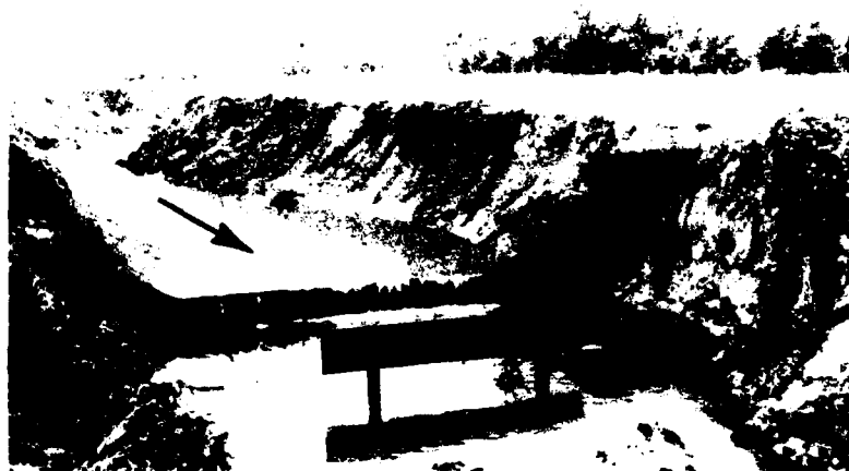
Exhibit XI-7. Typical grade-control structure, Johnson Creek. (Scour hole to be formed by hydraulic action)
