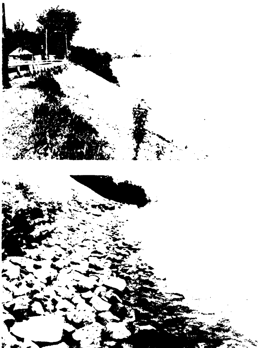
Exhibit XIII-4. Ohio River (left bank) at Cloverport, Kentucky. Downstream view shows toe of revetment under wave attack due to passing barge traffic (19 June 1978). Typical riprap revetment constructed by the Corps of Engineers (successful)
