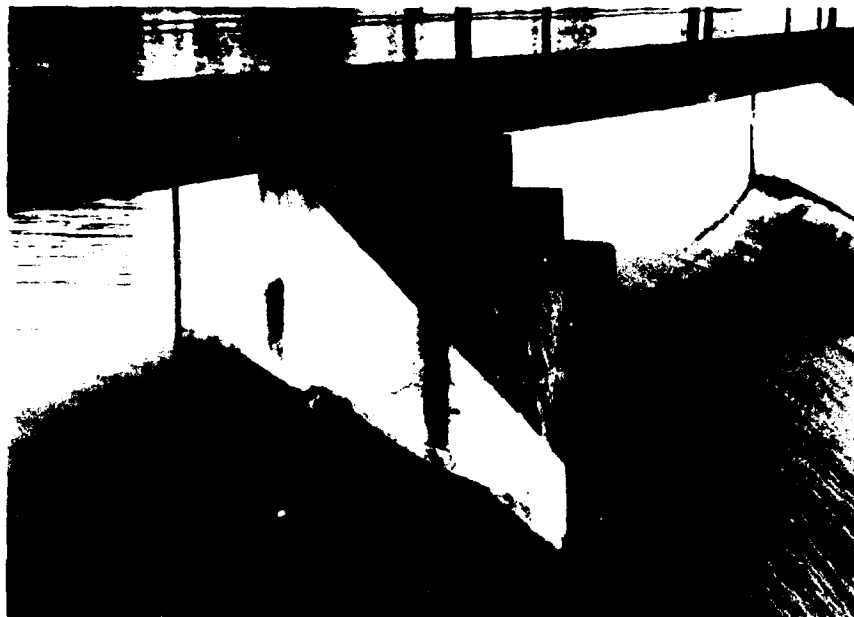
Photo 14. Taken from same location as Photo 12. Close-up of spillway pier No. 1. Boring D WES D7-80 was drilled through pier.
