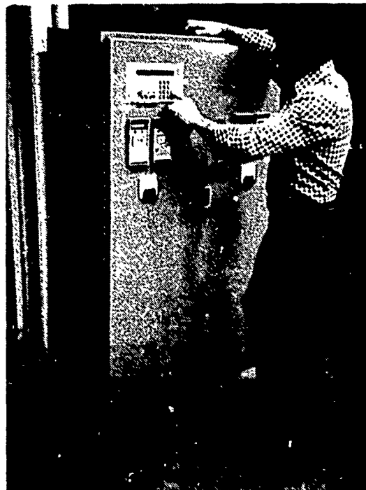
Figure 15. Barber-Colman microprocessor power control unit.
