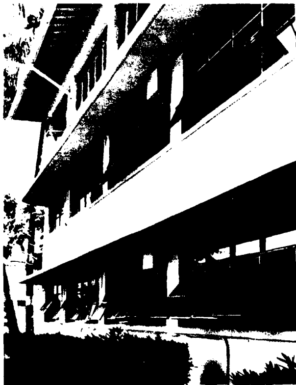
FIGURE 2 Protective Eave and Eyebrow Over Windows
