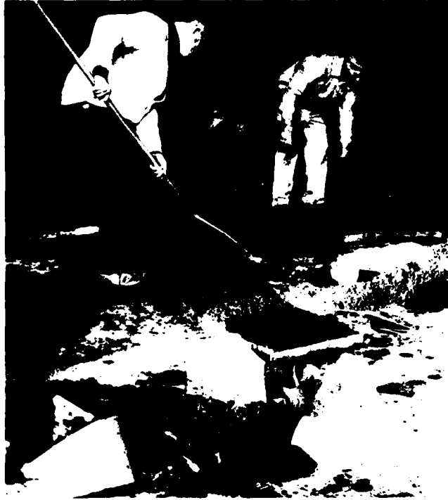
Figure A1. Raking dense-graded asphaltic concrete in the rolled aluminum angle forms for the circular track test sections.
