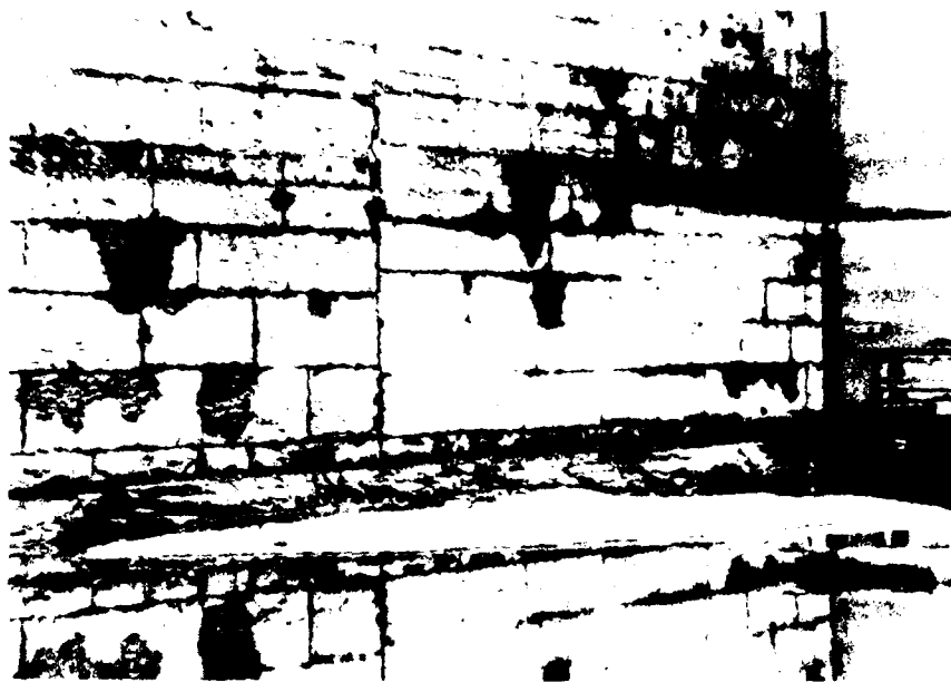
Photo 21. View of dry dock area at the Kankauna Project Office. Downstream of wooden gate showing masonry construction of wall founded on horizontal rock foundation
