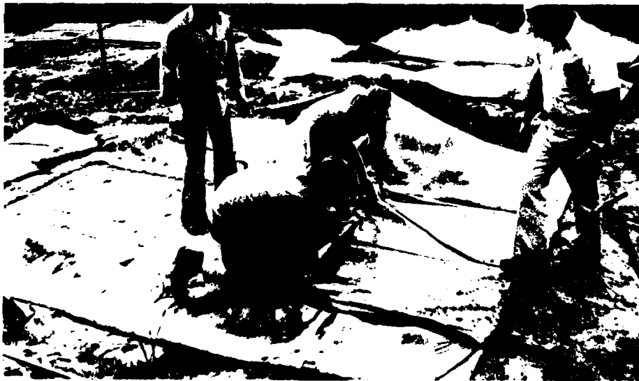
Photo 10. Closing flaps of membrane layer (nailing membrane to plywood)
