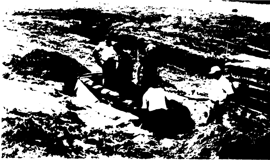
Photo 13. Upper support layer with sandbag form in place
