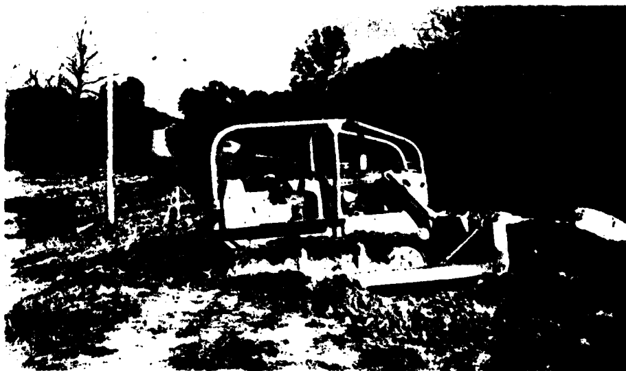
Photo 22. Cutting south approach
