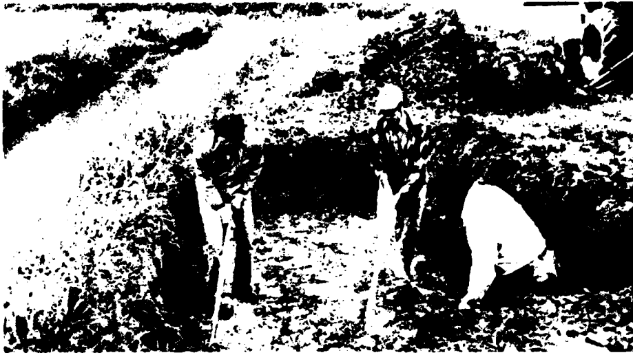
Photo 5. Finishing bottom of excavation
