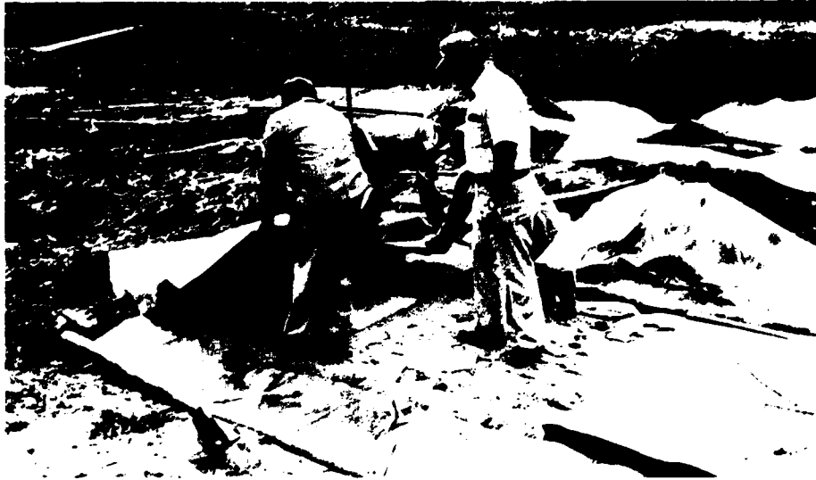
Photo 11. Closing flaps of membrane support layer (note plywood board)
