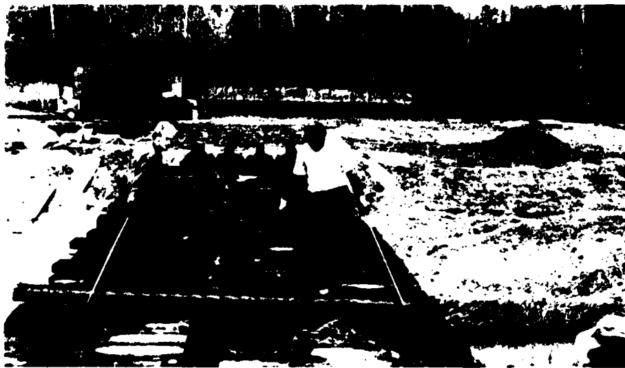
Photo 21. Placing decking on stringers
