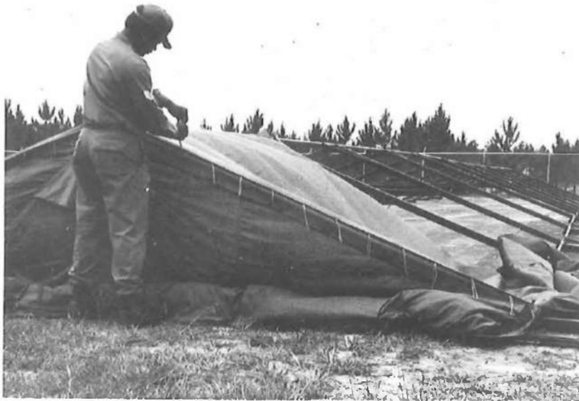
Figure 27. Beginning the Becket Sequence at Arch Ridge
