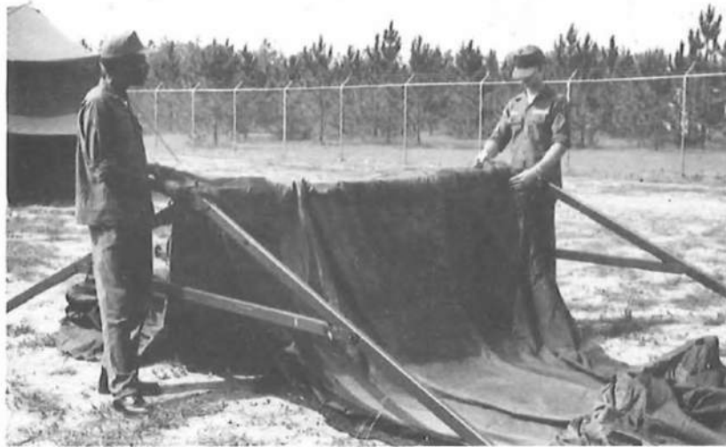
Figure 26. Roof Blanket Draped Across Frame
