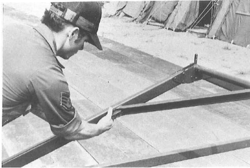
Figure 24. Purlin Brace Handle Properly Locked
