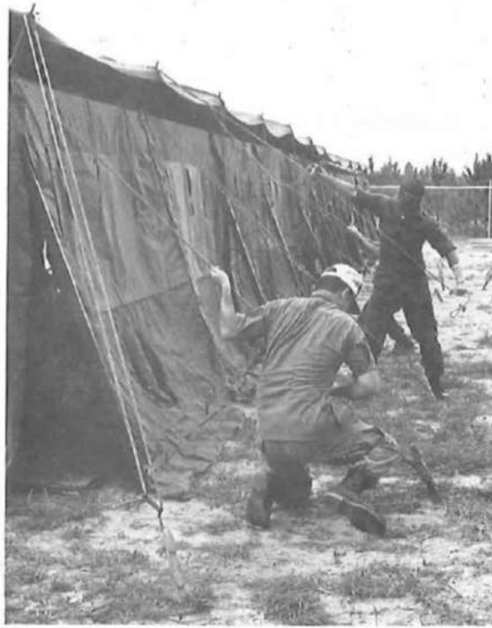
Figure 45. Attaching Guylines to Stakes
