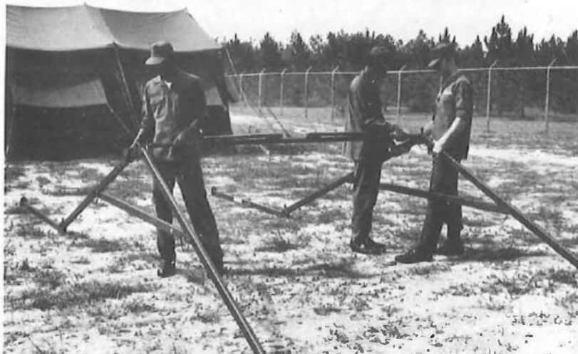
Figure 21. Standard Purlin Installed at Ridge
