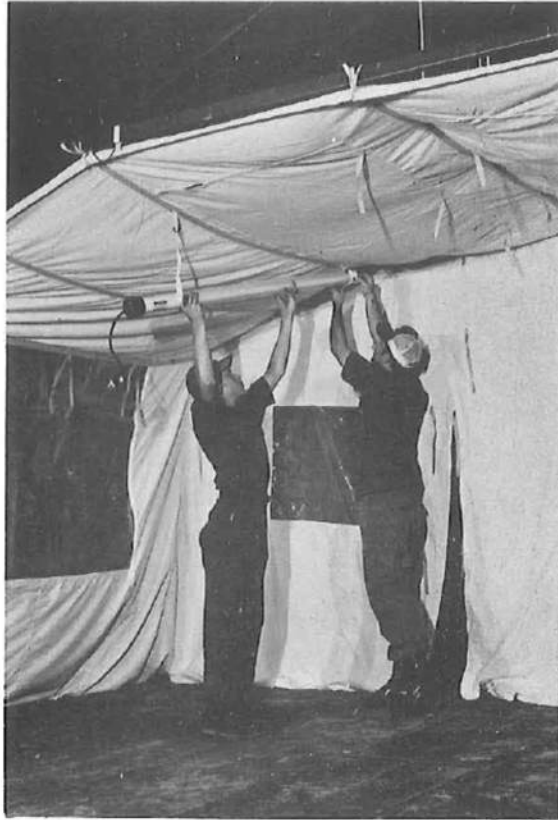
Figure 101. Lighting Tube Installation
