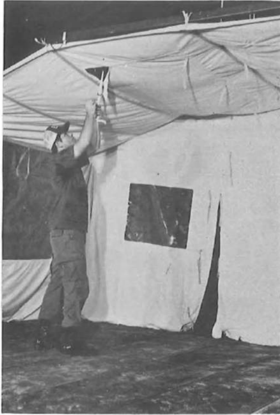
Figure 100. Lighting Support Strap Pulled Through Kitchen Liner
