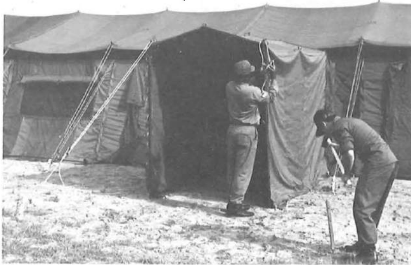
Figure 52. Securing Vestibule End (Freestanding)
