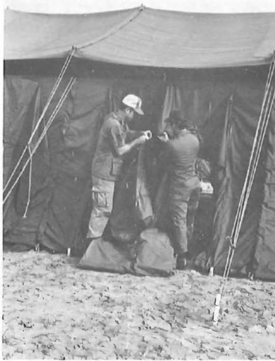
Figure 49. Becketing Vestibule Cover to Transition Piece
