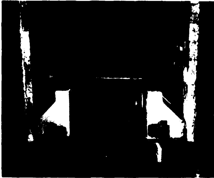
Figure 8 PIGS BEING DEPOSITED IN DECONTAMINATION FURNACE
