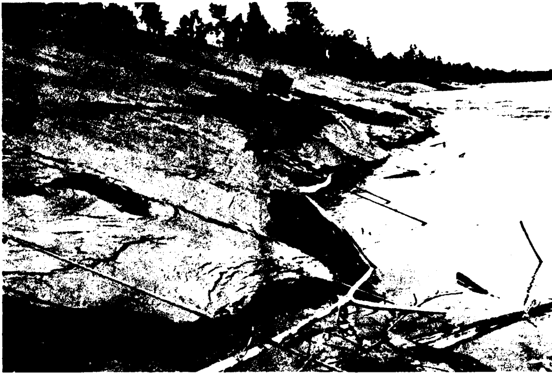
Figure 37. Failure of bituminous mattress
