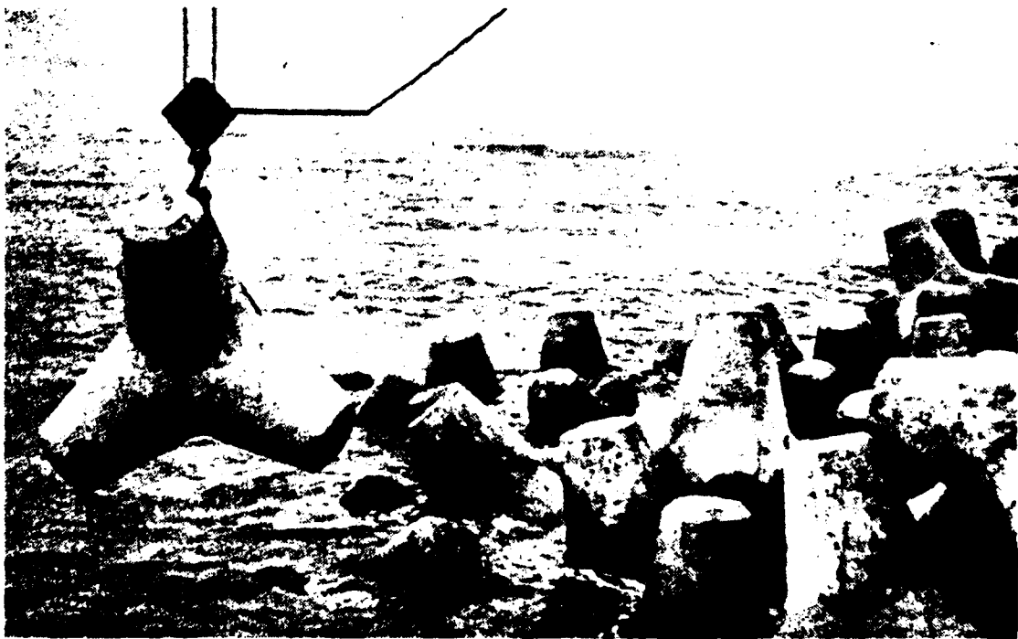
Figure 61. Tetrapods (photo courtesy of California Department of Transportation)
