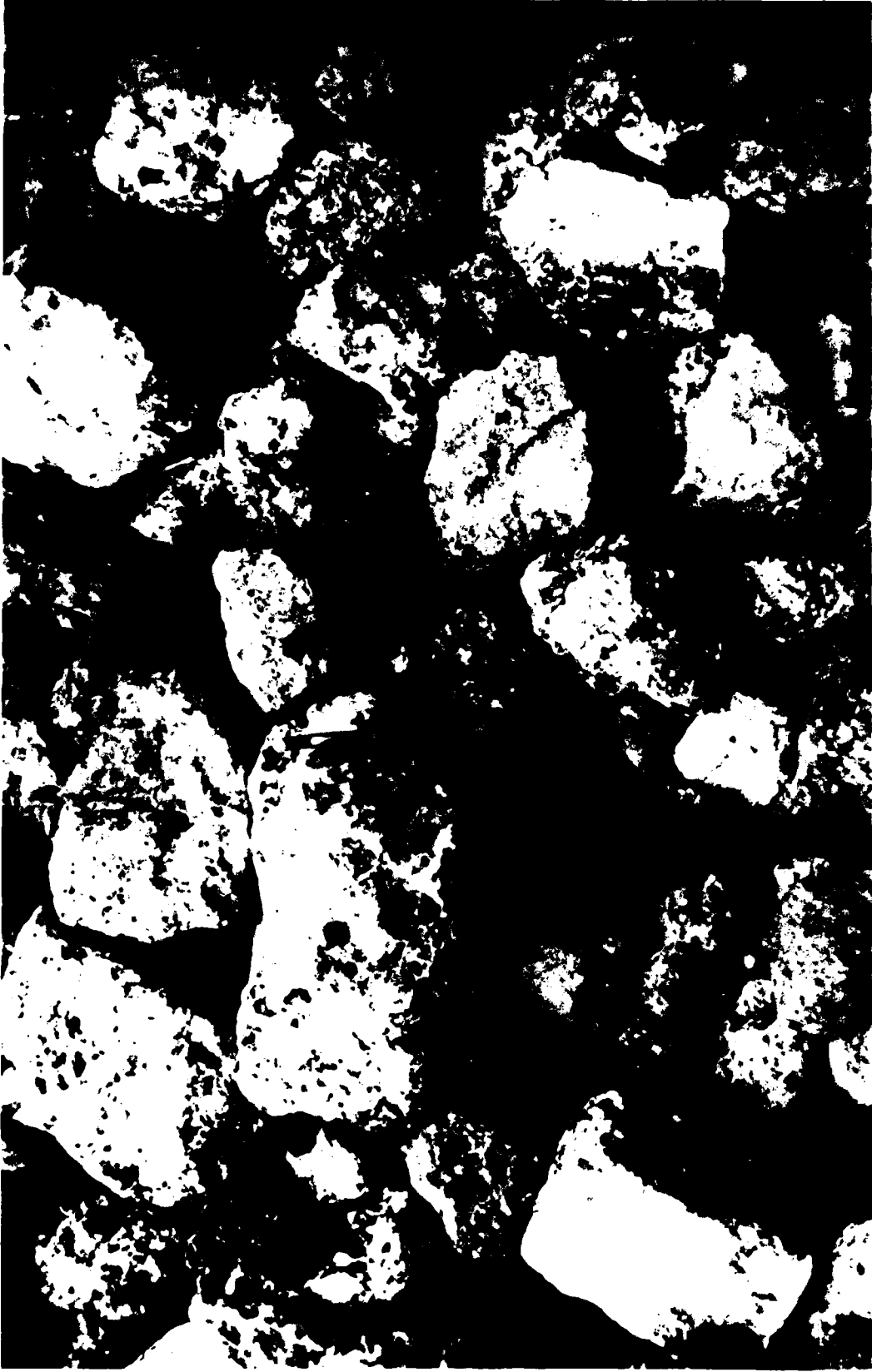
Figure 3. Detailed view of slag used to construct revetment
