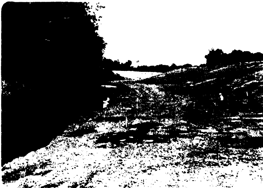
Figure 9. Clay blanket placed on the berm and lower portion of the side slope prior to seeding
