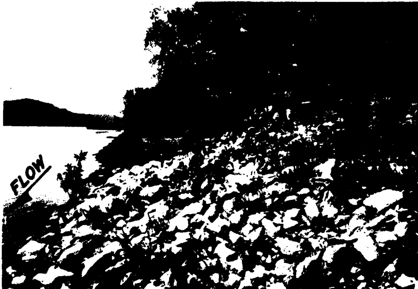
SCHEME B: LOOKING UPSTREAM AFTER CONSTRUCTION
