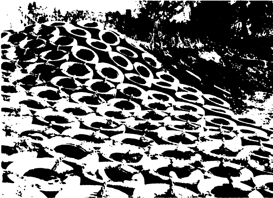
SCHEME C: LOOKING UPSTREAM DURING CONSTRUCTION
