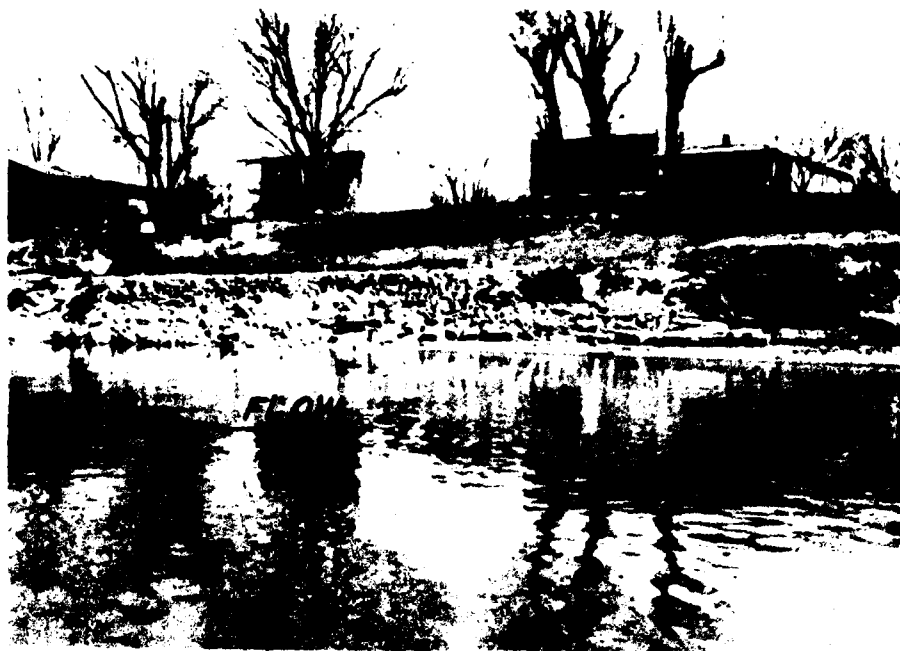
SCHEME C: LOOKING UPSTREAM BEFORE CONSTRUCTION
