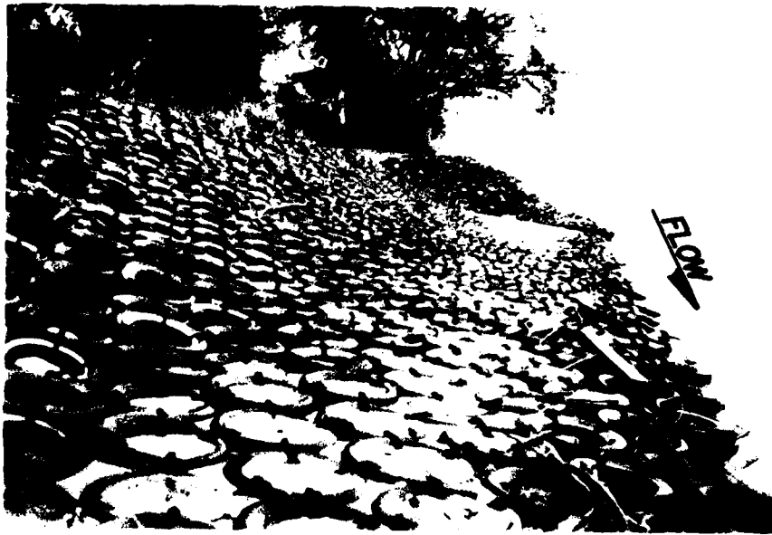
SCHEME C: LOOKING UPSTREAM AFTER CONSTRUCTION
