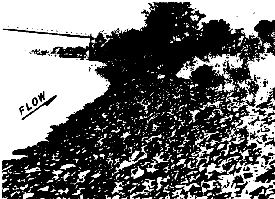
SCHEME D: LOOKING DOWNSTREAM DURING CONSTRUCTION
