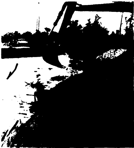
DURING CONSTRUCTION FROM STATION 21+00 12 MAY 1978
