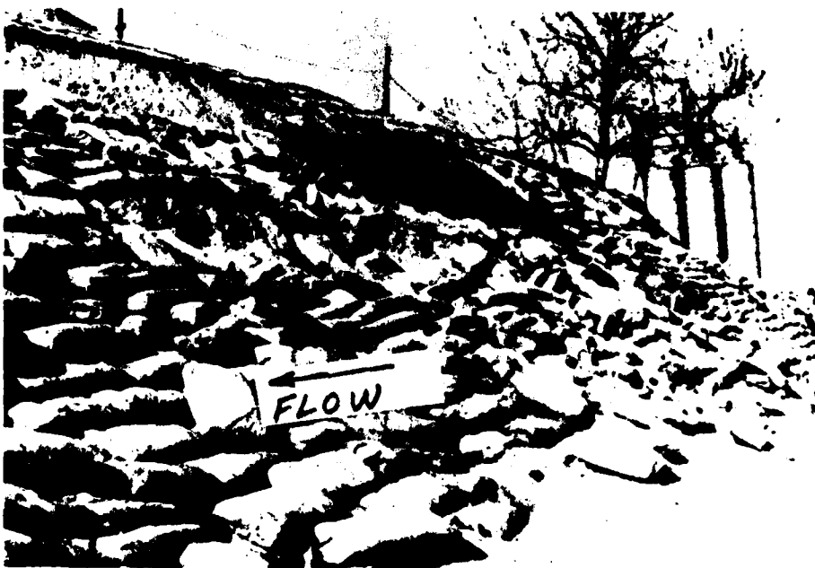
PHOTO NO. 8. May 79. Continued loss of cement bags due to loss of bedding material and sliding during high water. Rehabilitation obviously needed at that time.
