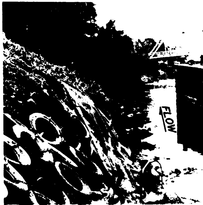
SCHEME A: LOOKING DOWNSTREAM DURING CONSTRUCTION
