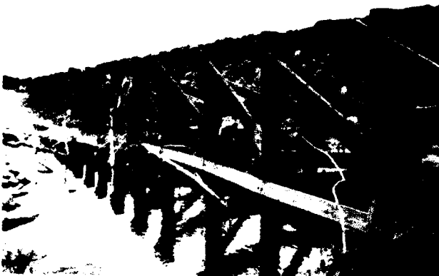
TIMBER PILE REACH
