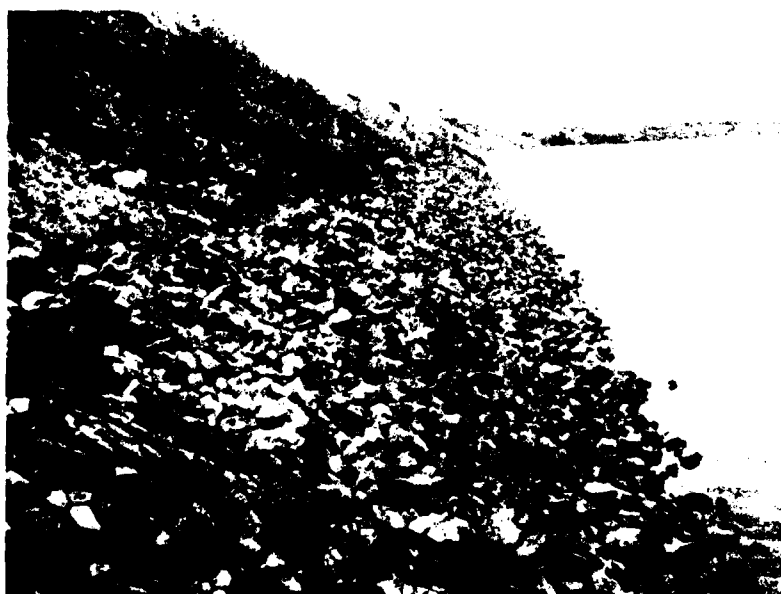
PHOTO 4 REACH 2A JULY 1979
