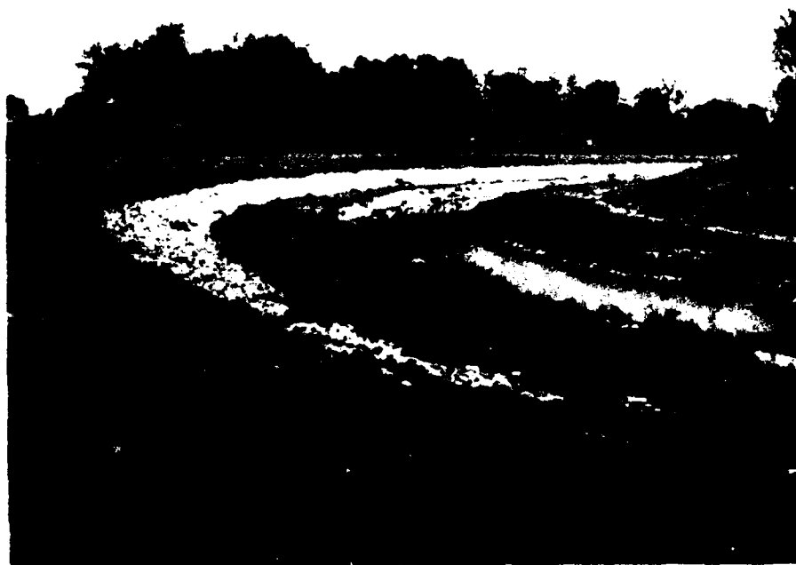
Figure 3. Little Blue River at Independence, Mo. Side slopes of low-flow channel protected by stone riprap
