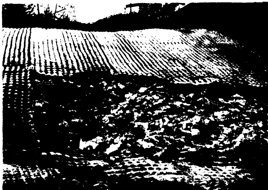
Figure 15. 102 River (East Fork) at Bedford, Iowa. View of damaged Fabriform revetment upstream of the State Street Bridge.
