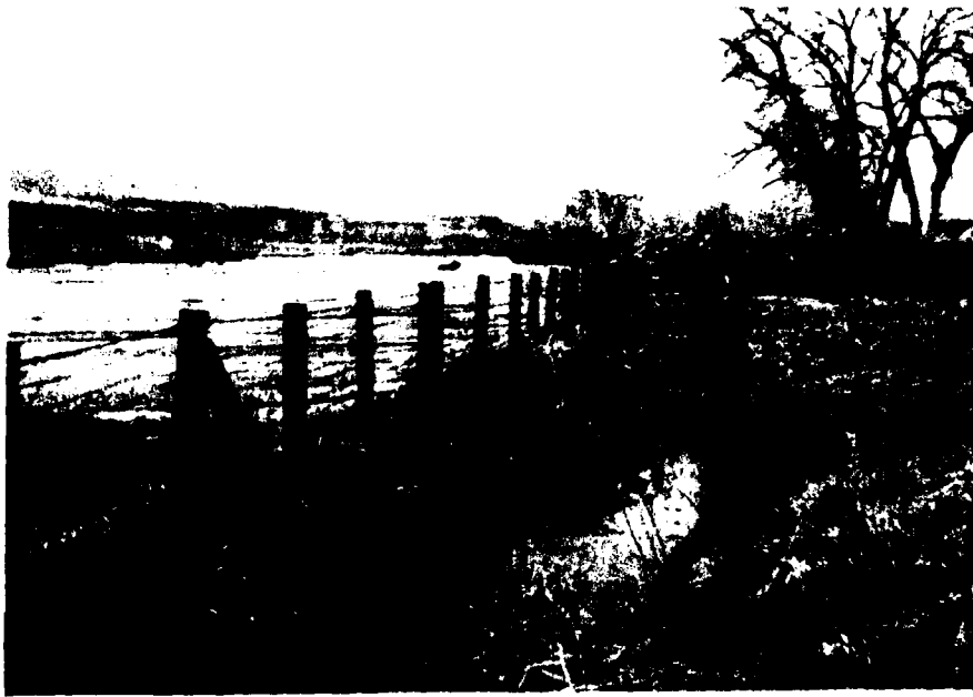
Figure 5. Plum Creek, Douglas County, Colorado. Landward side of fence revetment with tieback.
