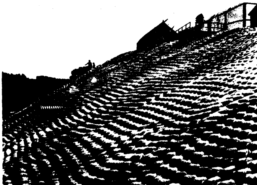
Figure 9. 102 River (East Fork) at Bedford, Iowa. Com- pleted Fabriform revetment at Bedford Sewage Treatment Plant.
