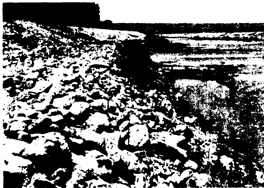
Figure 7. Republican River at Milford Dam Outlet Channel, Kans. Typical view of the revetment toes as of July 1981. Note break in slope between the blanket and the slope to the water.
