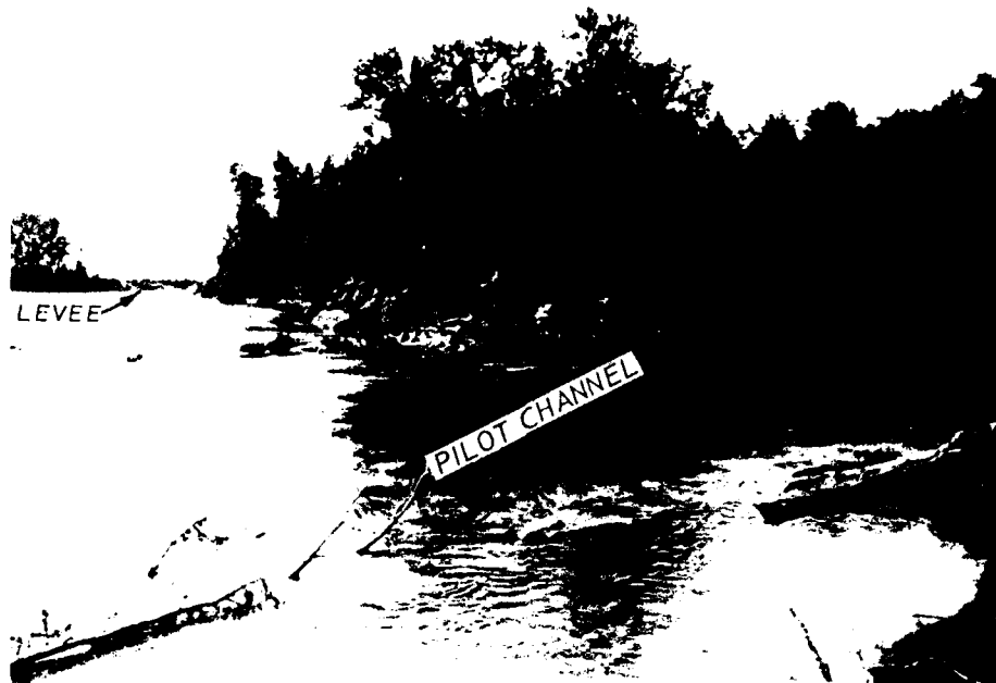
Pilot Channel 1, White River, Levee Unit 8 at Edwardsport, Inc. The upstream end of the pilot channel is to the right; the natural streambed is to the left. Note the levee in the background and deposition in the natural channel. The estimated total discharge is approximately 5,600 cfs, with 95 percent flowing through the pilot channel (20 June 1978). View toward downstream direction
