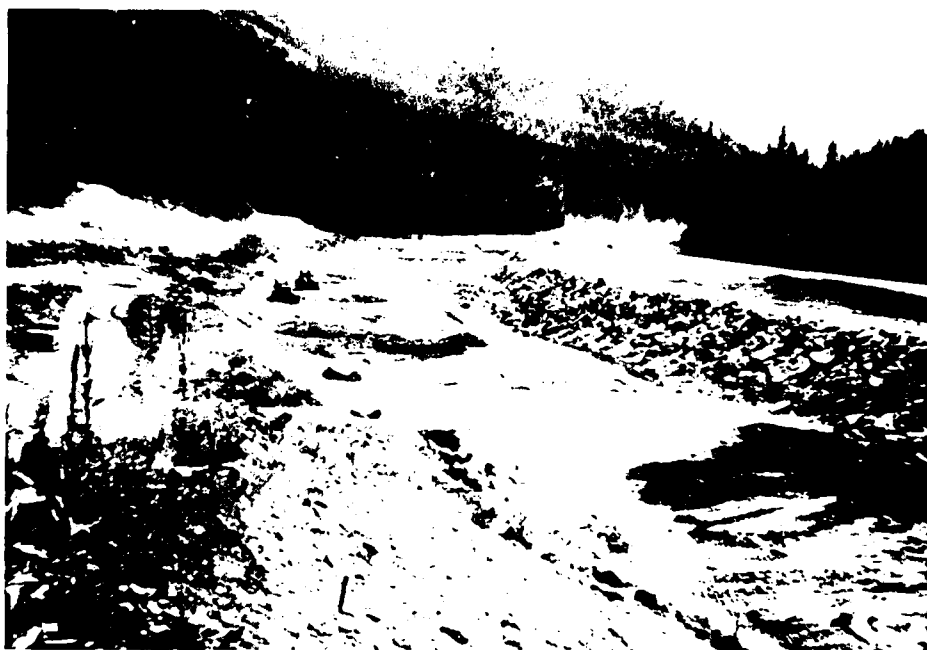
a. Under construction (24 Aug 67)
