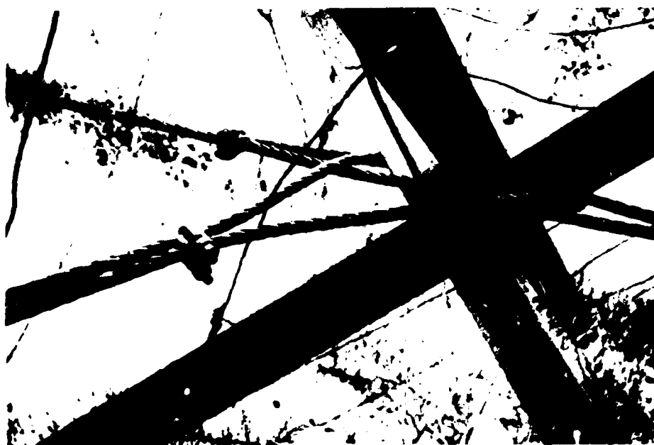
Jacks units are connected with steel cable; this figure shows the cable configuration at the junction of a main-line jetty and retard line
