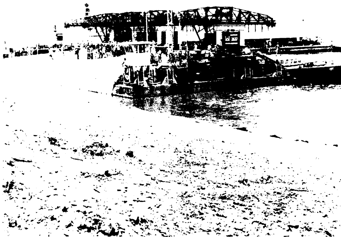
Figure 51. Articulated concrete mattress sinking operation (Launching barge is at left; from Keown et al. (1977))
