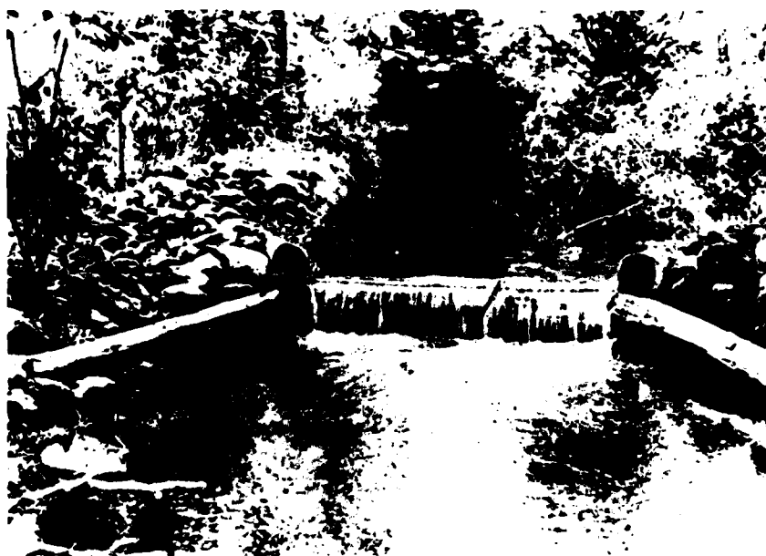
Figure 25. Hewitt ramp (This log barrier made of securely anchored logs scours a pool at its downstream face; photo courtesy of the Minnesota Dept. of Natural Resources.)
