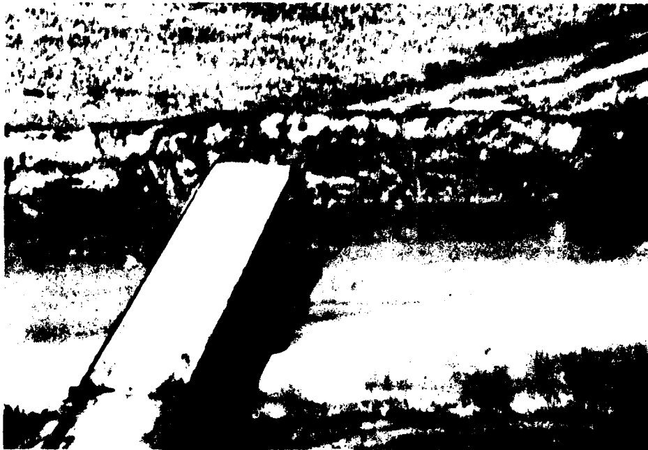
Figure 15. Bridge crossing destroyed by unstable channel widening (The site shown here is upstream of a channelized reach of Twenty-Mile Creek, Miss.; photo courtesy of the U. S. Army Engineer District, Mobile.)
