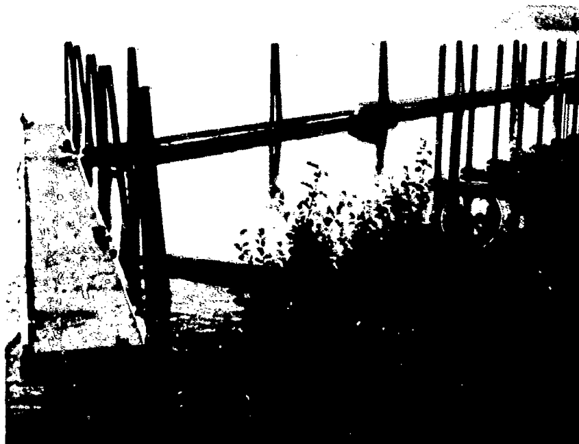
a. Floating breakwater section.
